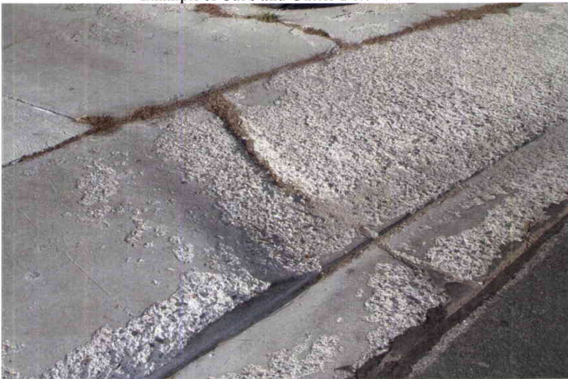
Example of Curb and Gutter Deterioration
