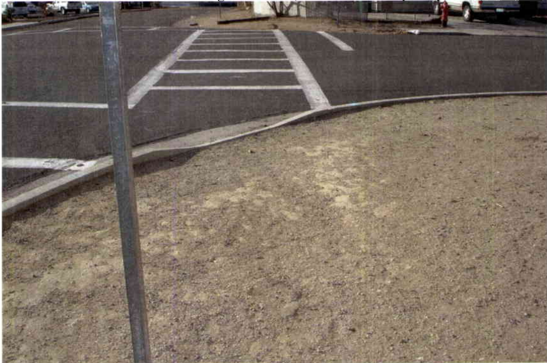
Crosswalk w/Curb Cut to Missing Sidewalk (at intersection by Empire Elementary)
