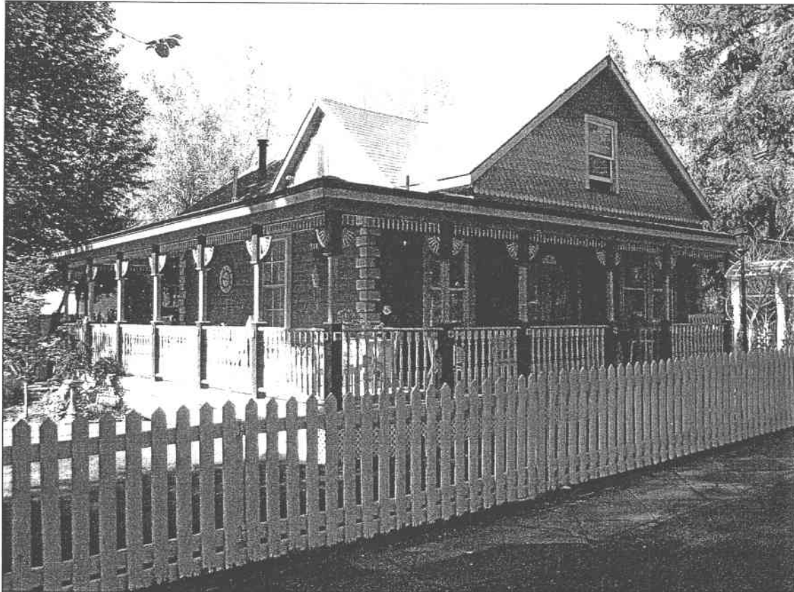
North and east facades
