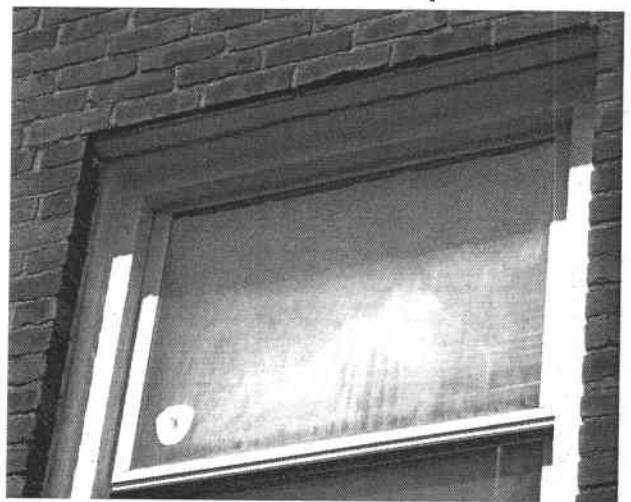
When the seal on insulating glass fails, the window loses its insulating properties and the glass fogs up. Photo courtesy of Paul Trudeau
