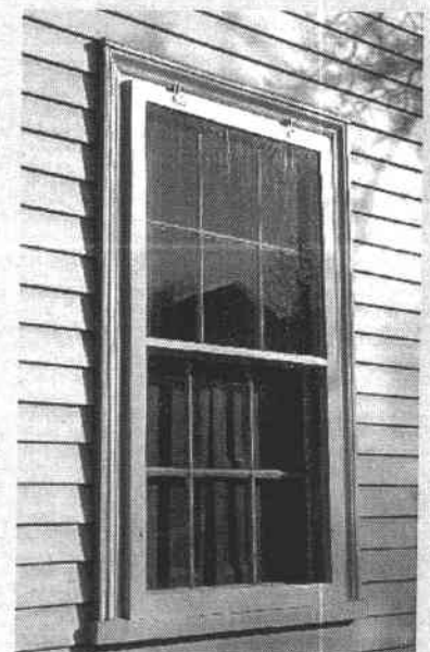
Storm windows that are installed flush within a window casing can have a minimal impact, as shown with this wood model. Image source: http://smithrestorationsash.com/woodstormwindows.html
