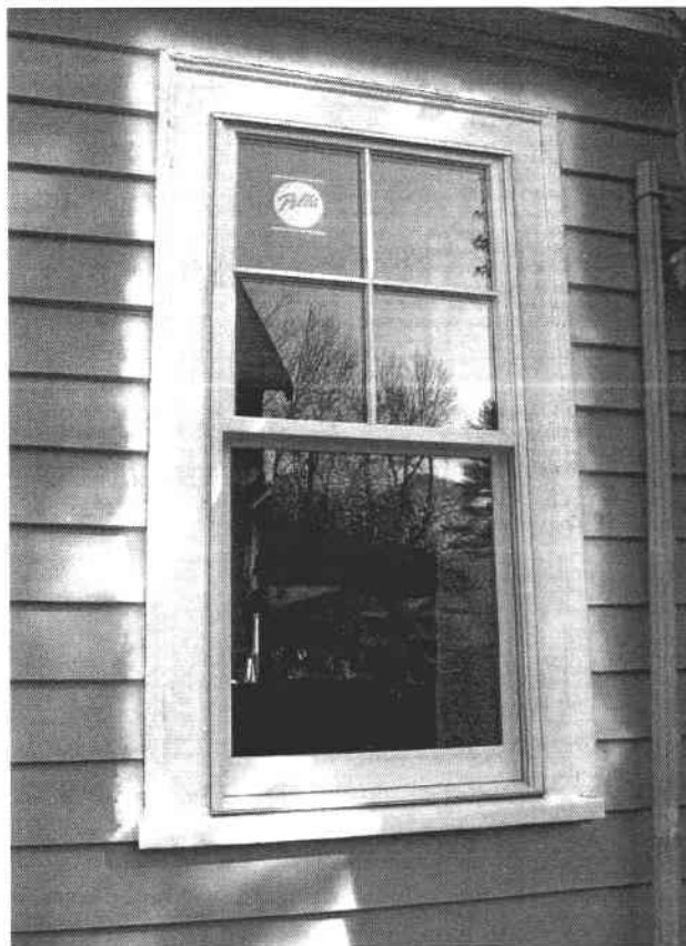
The framing component required for this replacement window model diminishes the window's rough opening by several inches. Photo courtesy of Paul Trudeau
