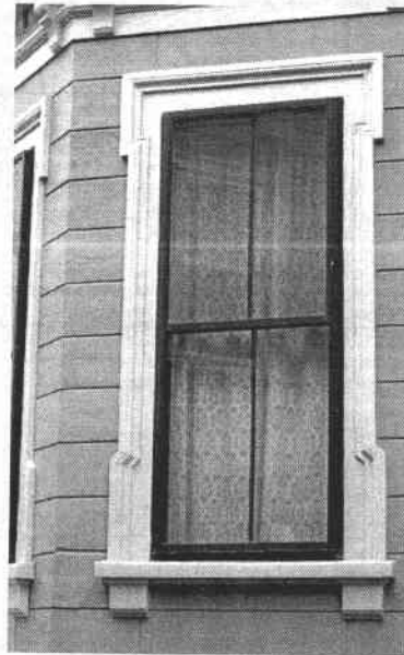
A quality aluminum storm window can be an appropriate addition to a historic window. Photo courtesy of Paul Trudeau
