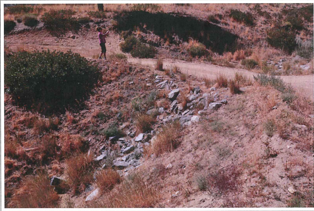
Photo 2. View of rock lined drainage near MP 1.2.
