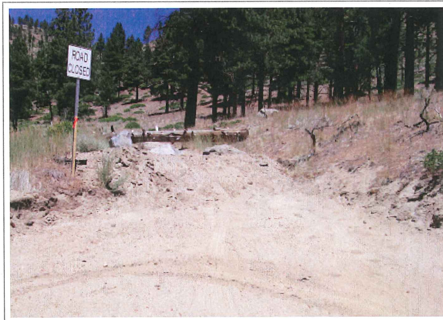
Photo 5. Road #2 closure with log, berm, and boulders near MP 1.65.
