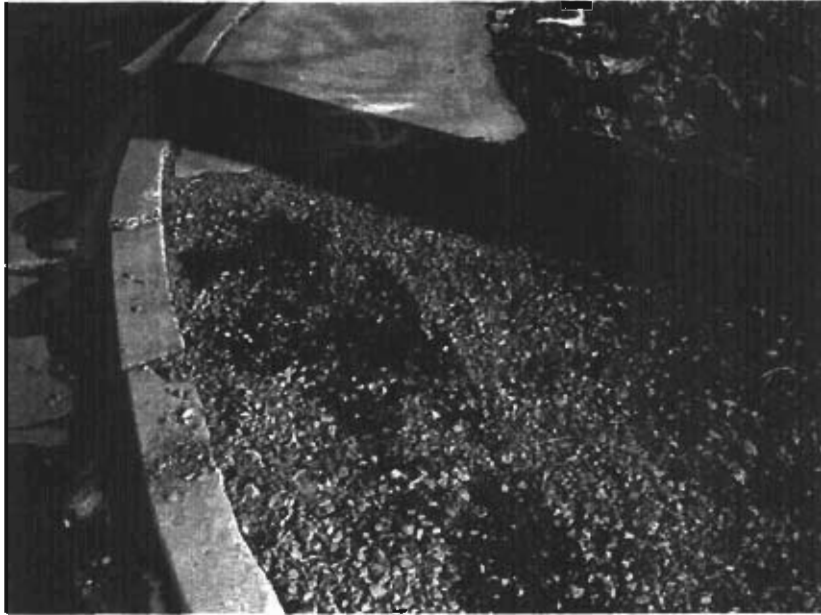
Deteriorated Sidewalk and Lack of Curb Ramp
