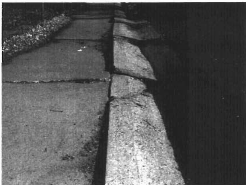
Tripping Hazard and Poor Drainage Due to Curb & Gutter Displacement
