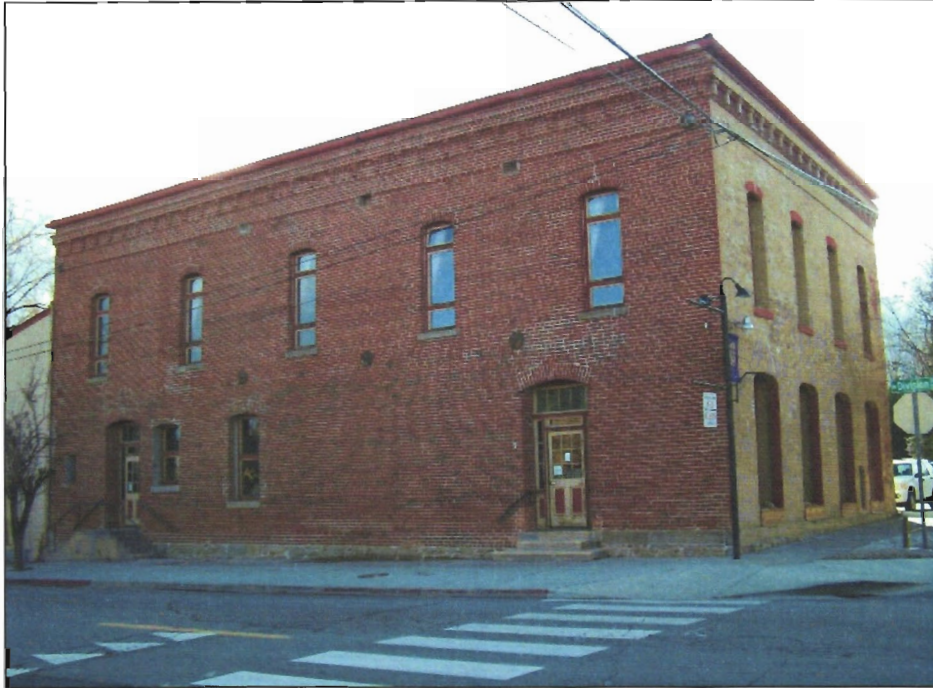
Carson City Parks and Recreation Department 449 W. King Street, Brewery Arts Center Project Year: 2010 Project Description: Brick Façade Renovations
