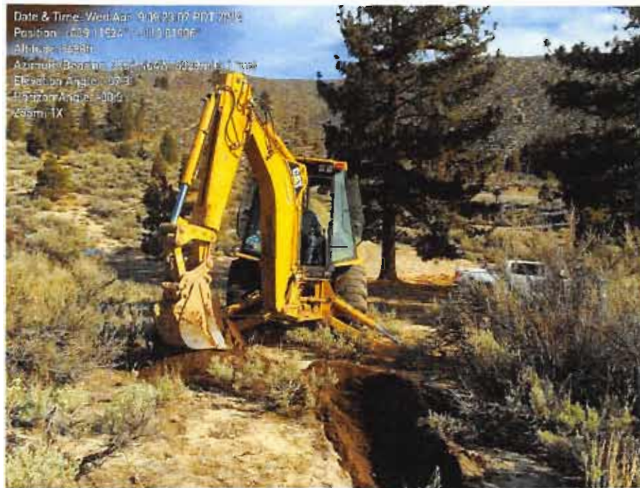
PHOTO 1 – Percolation Test Pit TP – 1.
