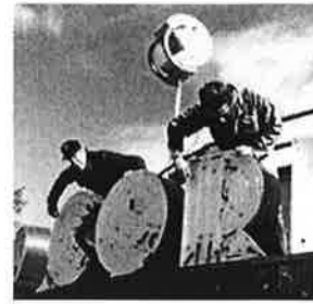
Neon fabricators are installing the new tubing in the repaired and remounted cans. Photo: Larry Kanter.
