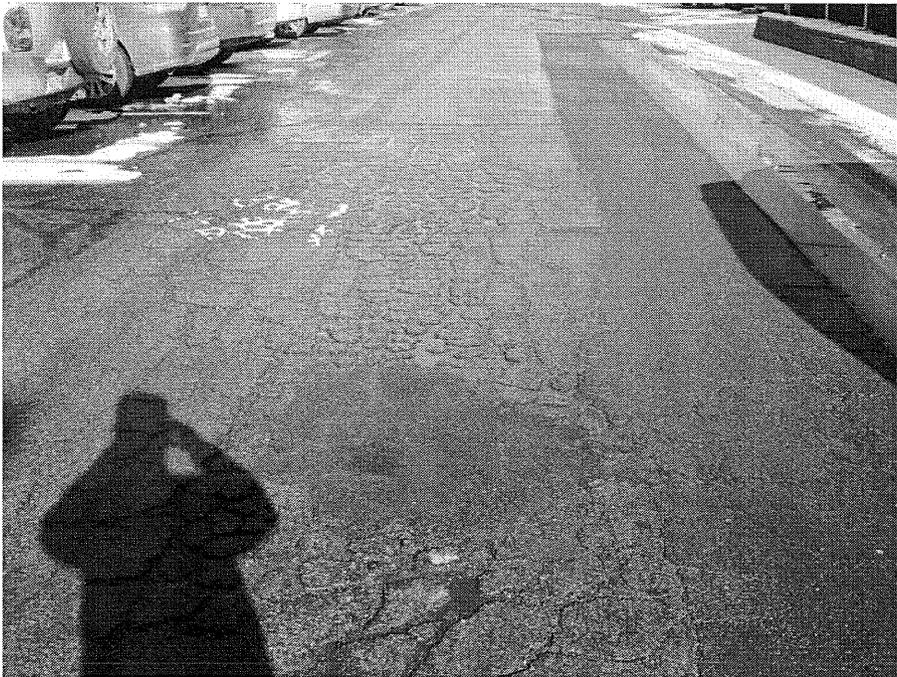
Alligator cracking and ponding in pavement
