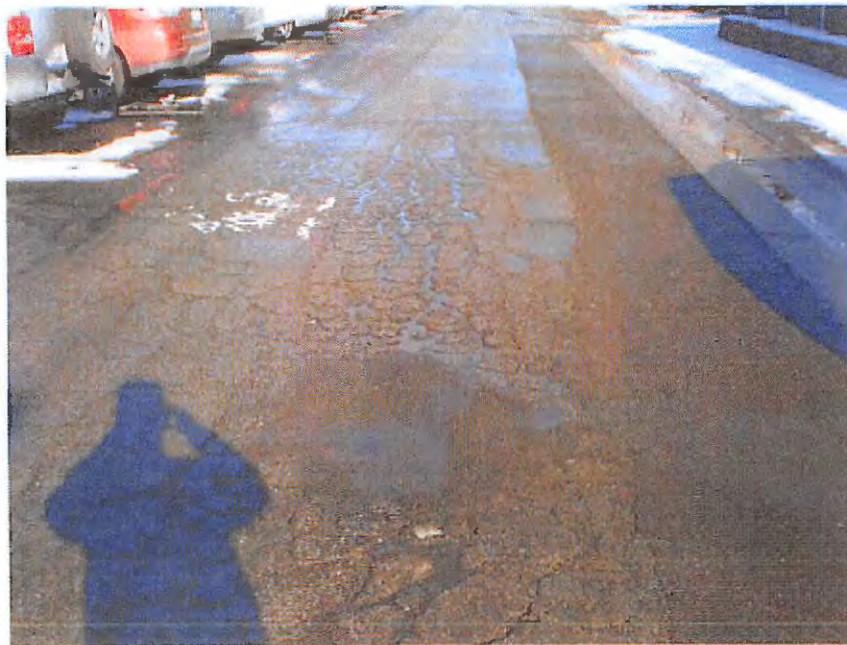
Alligator cracking and ponding in pavement
