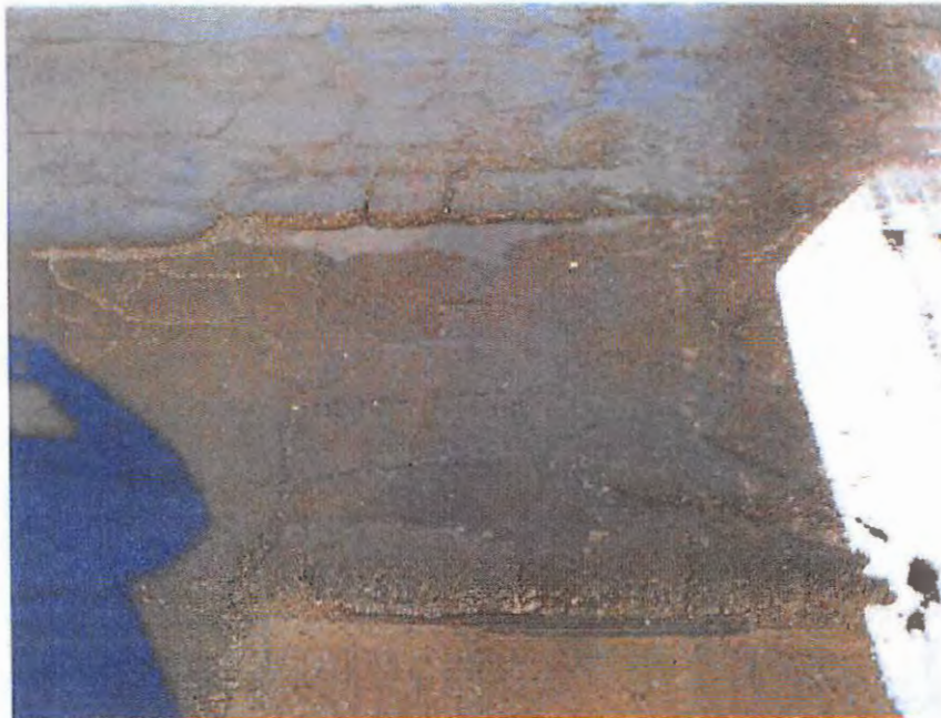
Pothole & ponding north of existing valley gutter
