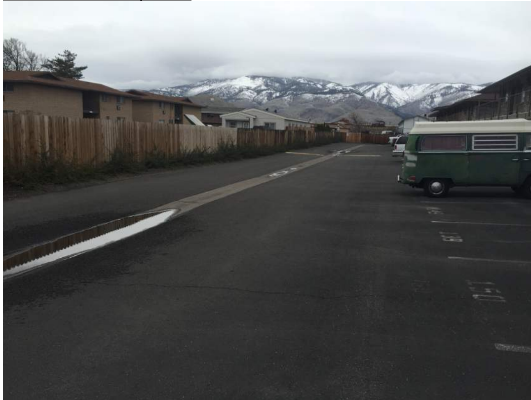
Water Pooled in Valley Gutter
