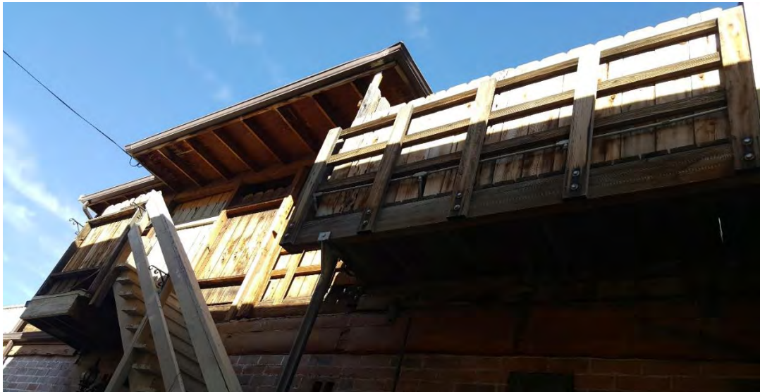
408 Carson Street – Alley side – Top floor and ground level floor
