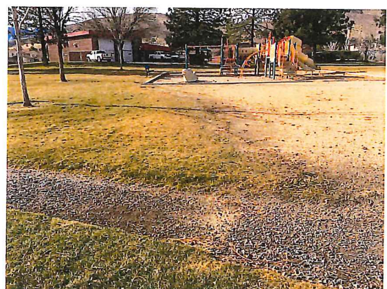
No existing accessible route to playground along path from stalls to playground. Path surface is not ADA compliant.
