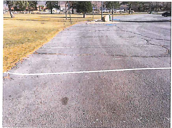
Non ADA compliant slope at location of existing and proposed accessible parking stalls.
