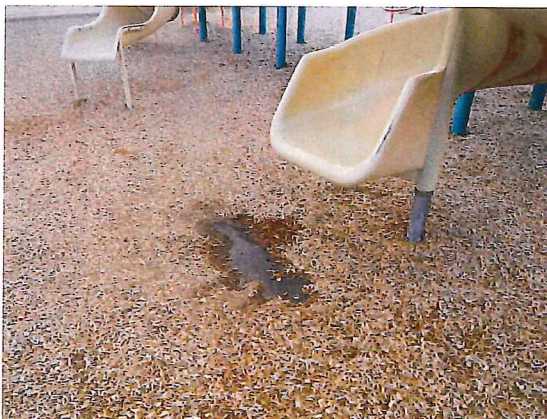
Existing playground surface conditions. Fibar surface showing movement of the material.
