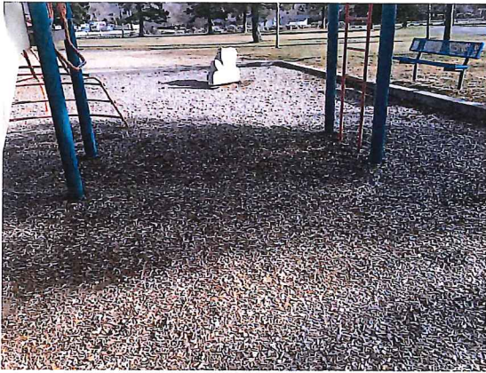
Existing playground surface conditions/ Fibar surface.
