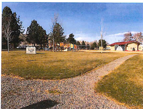
No existing accessible route to playground along path from stalls to playground. Path surface is not ADA compliant.
