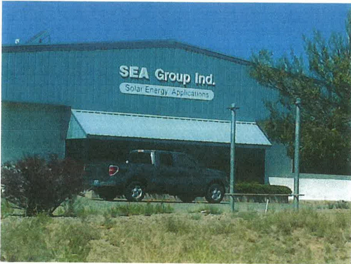
Photo 2 - Front Building Sign (facing east)
