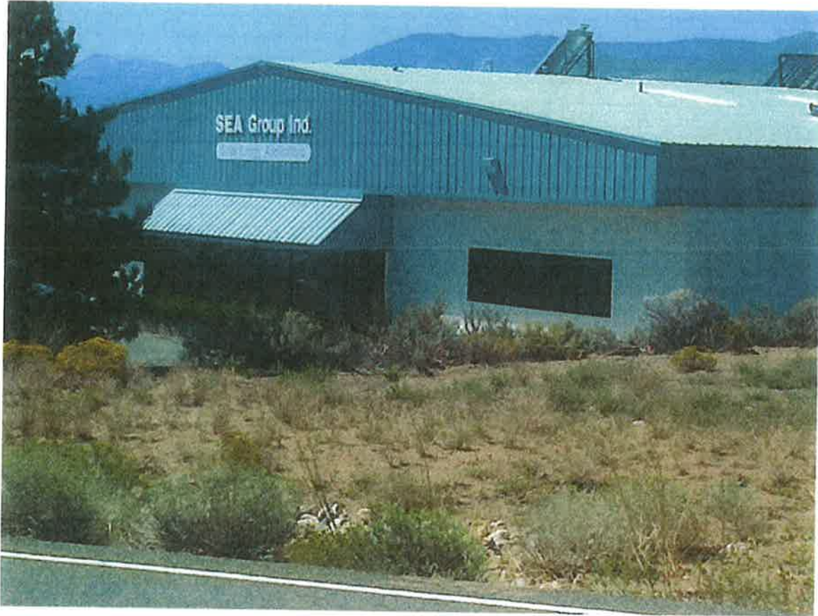
Photo 4 – Front Building Elevation (above the site)
