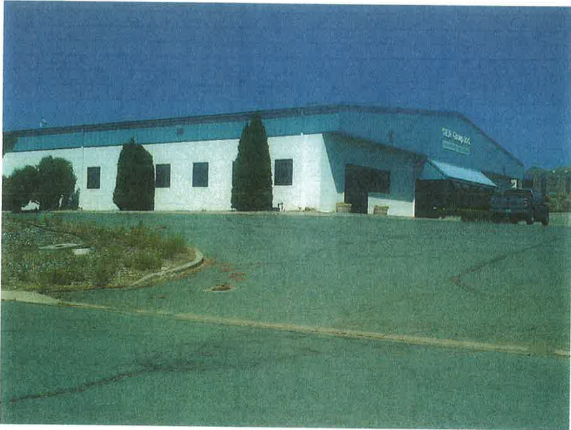
Photo 5 – Southeast Building Elevation (from Lamotte Road)
