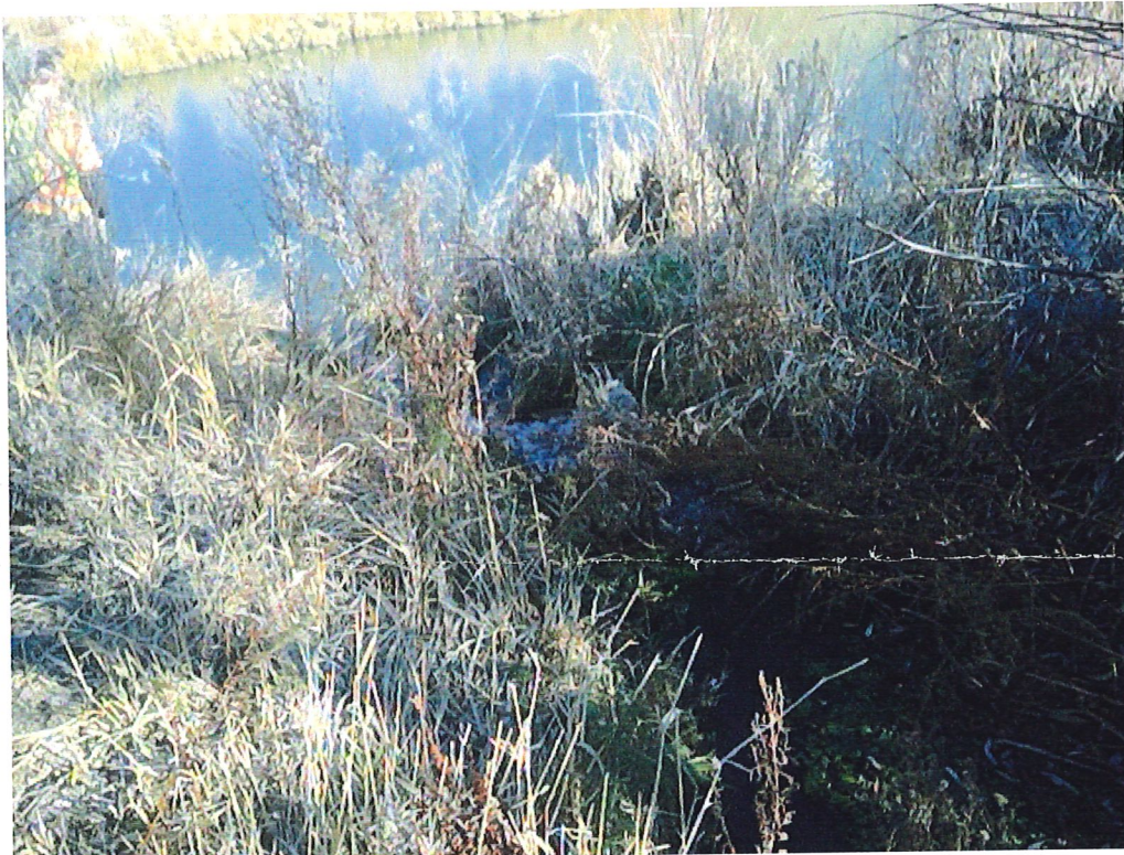
Seepage flowing into the Carson River.
