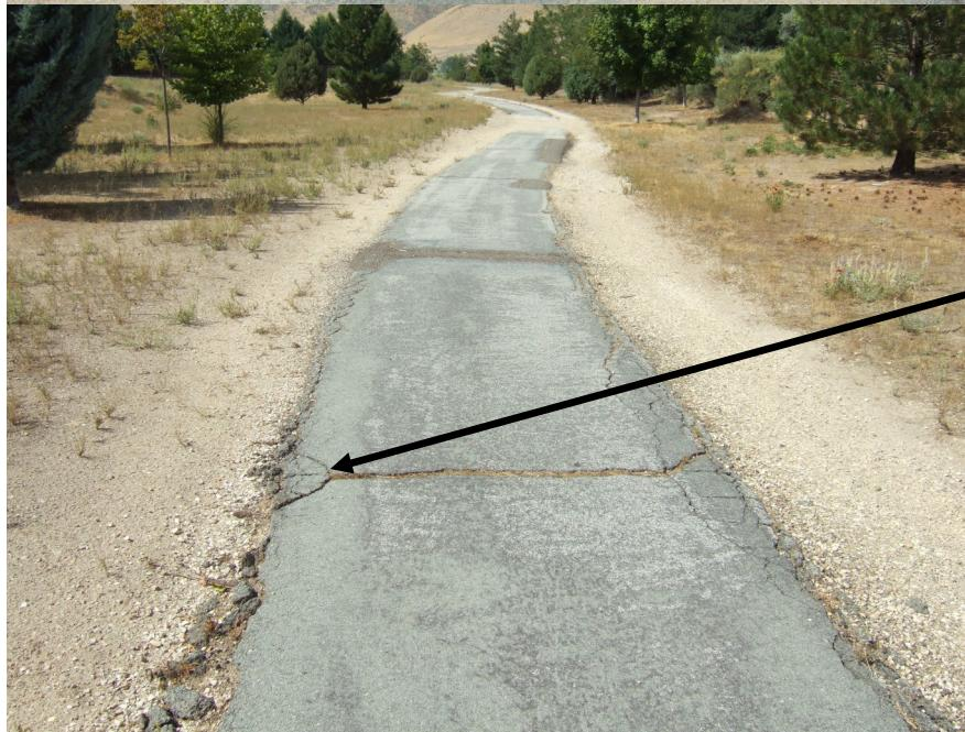
Edge of pavement is crumbling, severe bilateral cracks are forming, creating potential tripping hazards.
