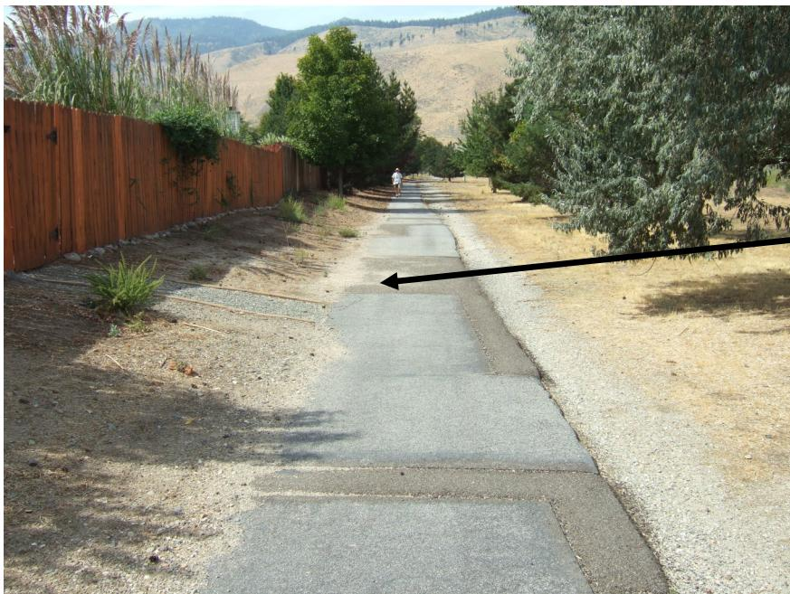
Gaps are forming at previous patched areas and drainage is impacting wear and maintenance.
