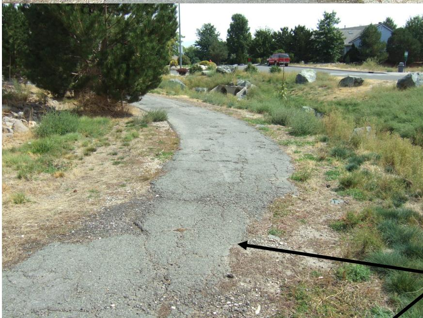
The path is deteriorating and crumbling in many locations, especially at curves, high use sections and transition points.
