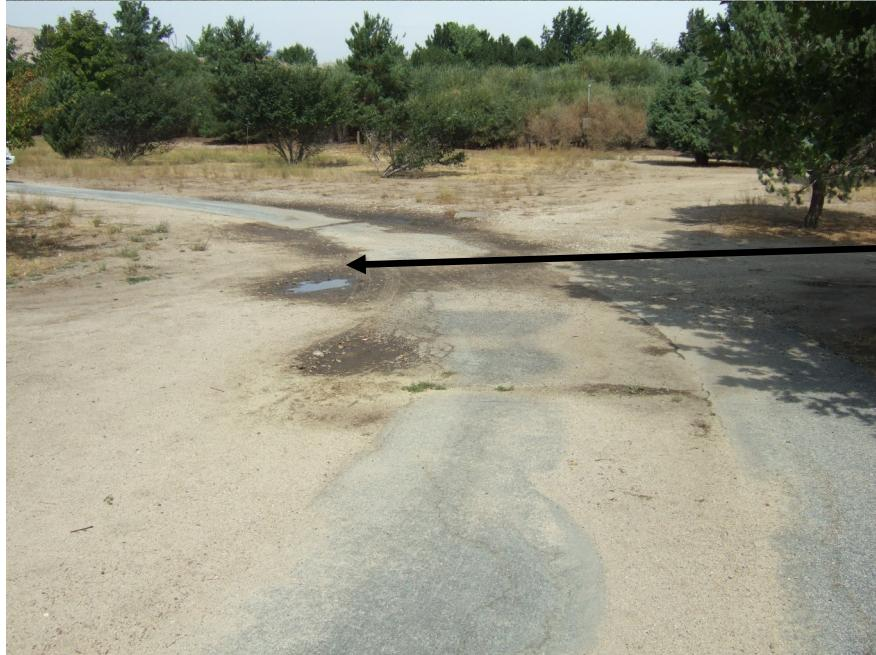
Impacts from cross slope and drainage are deteriorating the path, which impacts needs for on-going maintenance.
