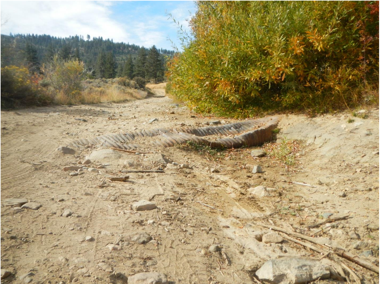
Photo 6: damaged and non-functional culvert.
