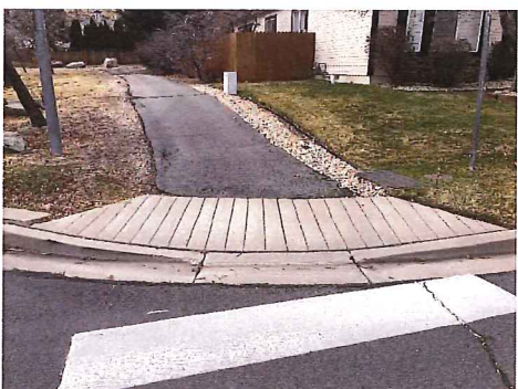
S SIDE OF BRISTOL PL AT THAMES LN INTERSECTION
