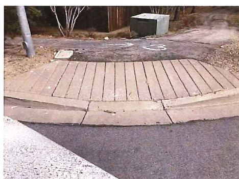
N SIDE OF LONGVIEW WY TURN-OFF FROM KINGS CANYON RD
