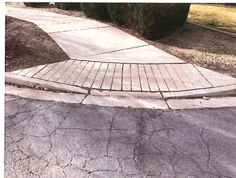
S SIDE OF WATERFORD PL AT THAMES LN INTERSECTION
