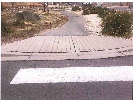
N SIDE OF WATERFORD PL, W OF INTERSECTION
