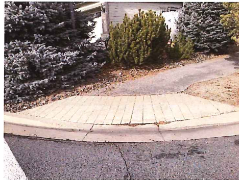
N SIDE OF WATERFORD PL AT THAMES LN INTERSECTION
