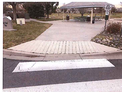
N CORNER OF BRISTOL PL AT LONGVIEW WY INTERSECTION
