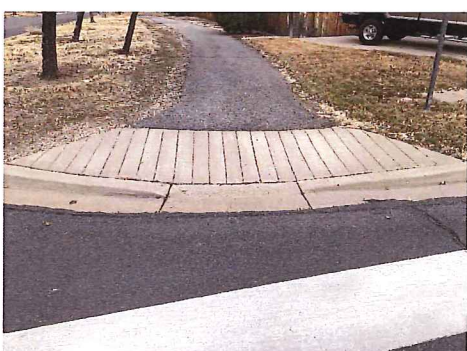
NE CORNER OF INTERSECTION AT ST GEORGE WY AND THAMES LN
