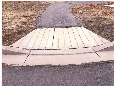
SE CORNER OF THREE-WAY INTERSECTION ON OXFORD CT AND THAMES LN
