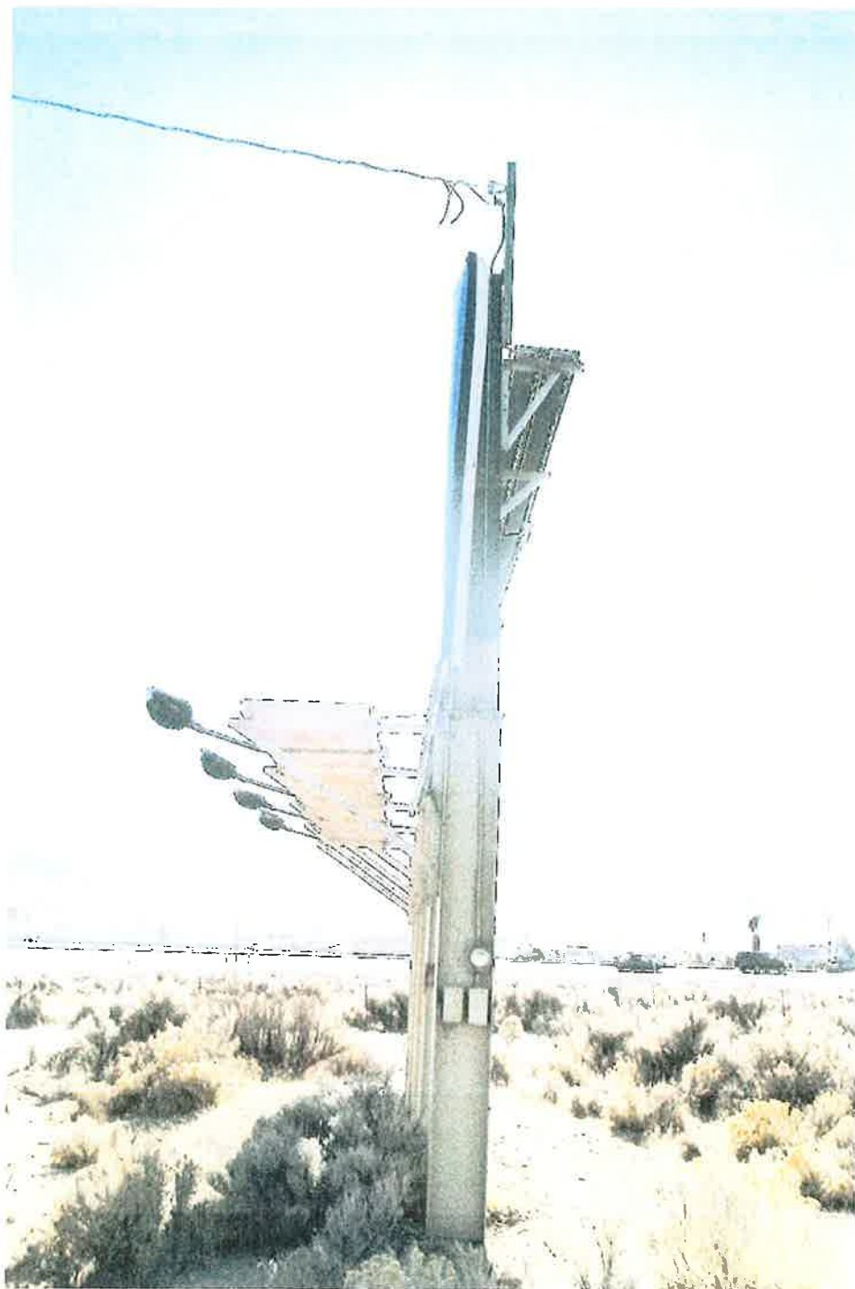
Side of Billboard showing power line, electrical panel and meter.
