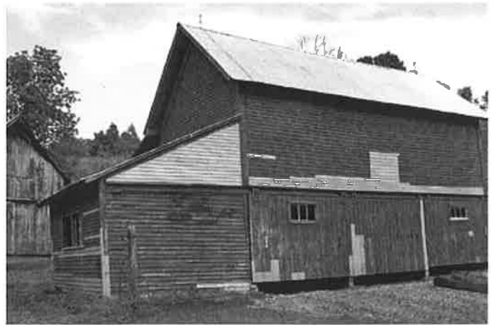
The siding on this barn was repaired with matching siding, a treatment that meets the Secretary of the Interior's Standards for Rehabilitation. Photo: Vermont Division for Historic Preservation.
