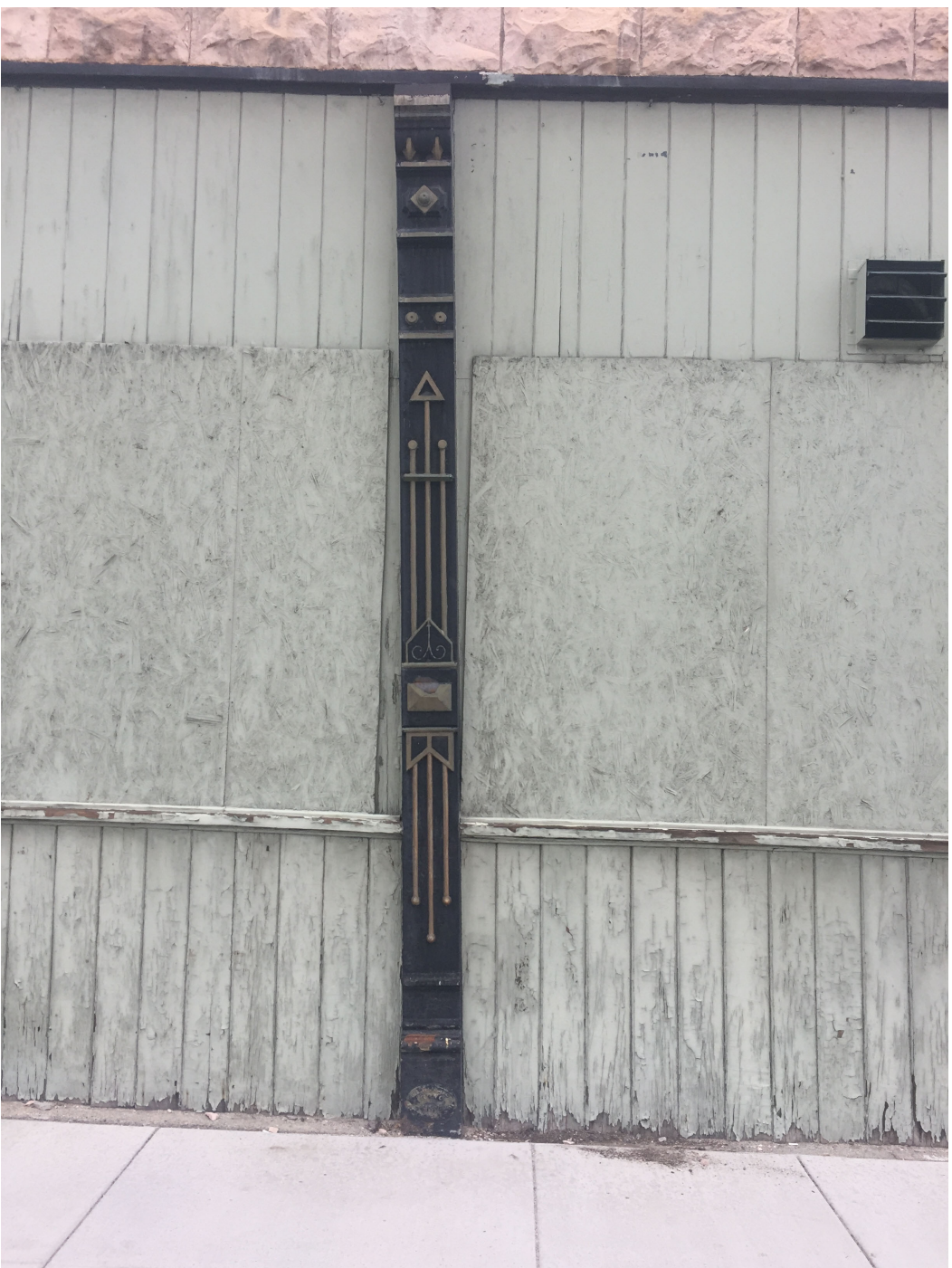
PHOTO 4 PILASTER BETWEEN WINDOWS
