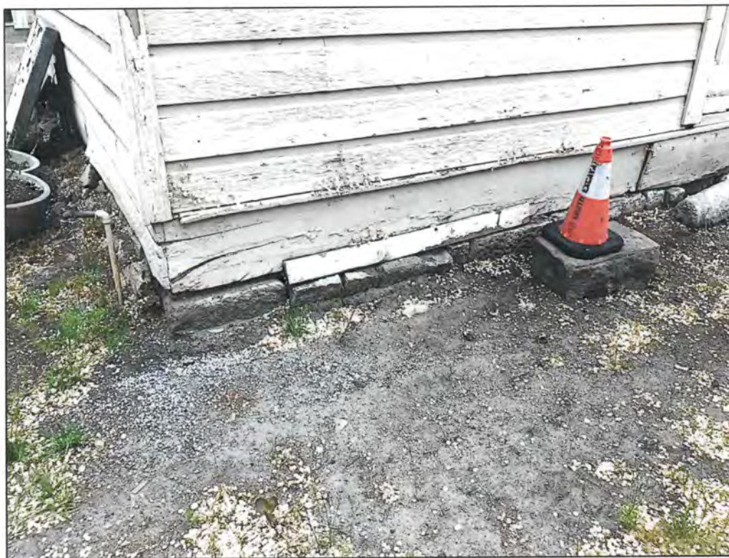
Figure 13. Curry House Outbuilding, sandstone foundation, looking southeast (Photo by Corri Jimenez, 2019).
