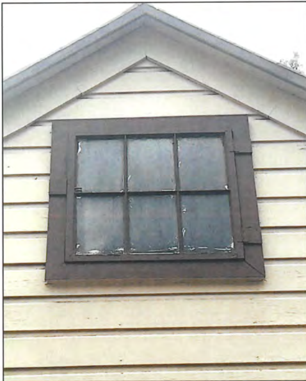
Figure 14. Curry House Outbuilding, looking at windows and doors. Top left: 1870s historic 4-panel door and transom; Top right: Door converted into a window with a vinyl window; Bottom right: 6-lite wood window in east gable end; Bottom left: covered 6/6 wood window on east elevation (Photo by Corri Jimenez, 2019).
