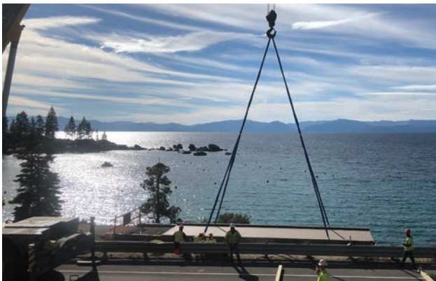
Crane placing fiberglass bridge deck.
