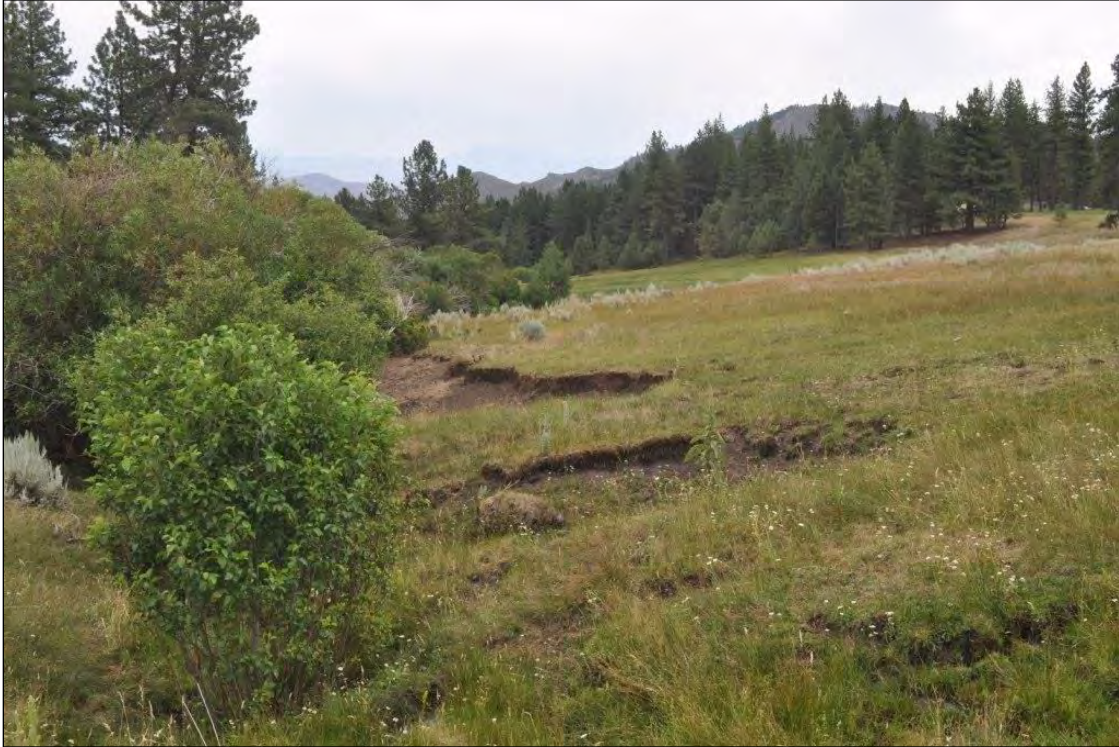
2013 Condition, photo taken July 23, 2013 (initial assessment – view south)
