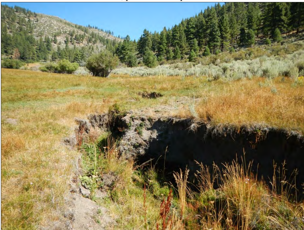
2019 Condition, photo taken September 12, 2019
