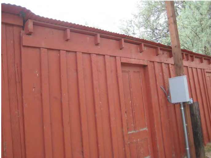
Board-and-batten siding and "barn red" color are architectural characteristics that define the complex
