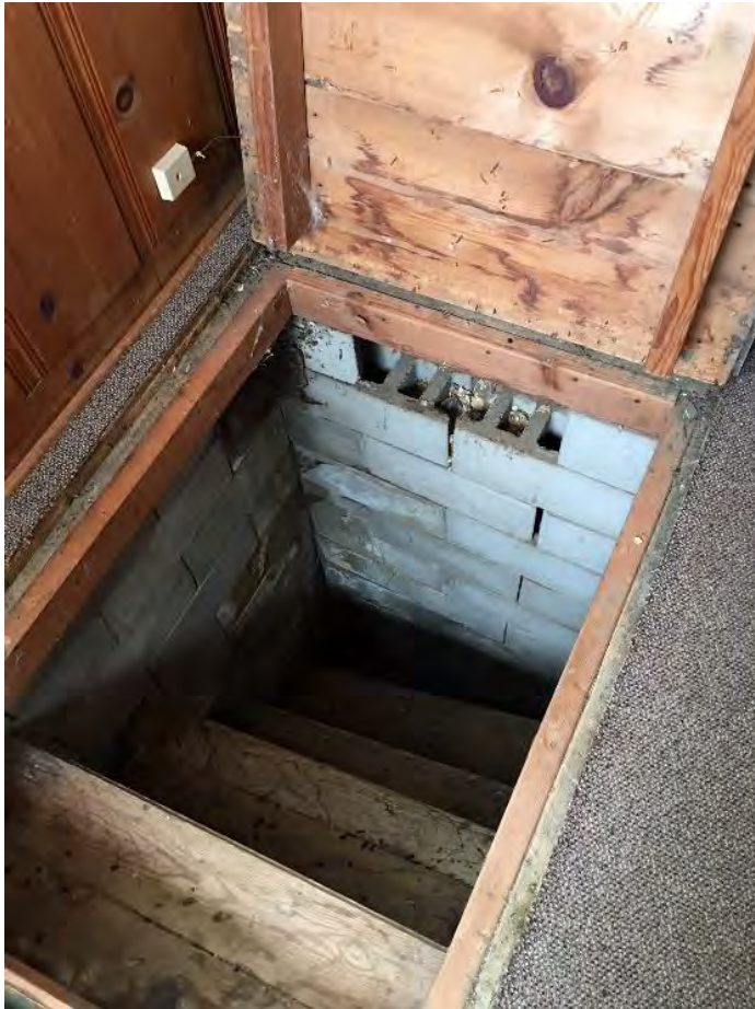
Floor hatch and staircase to cellar under the room in the hipped extension off façade of residence (possibly earlier open porch); note concrete block walls, no mortar visible in the open cells of the blocks suggesting an unreinforced masonry wall
