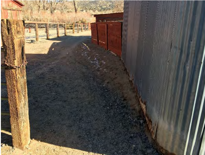
Top: Problem drainage at entry to ranch, metal in contact with earth
