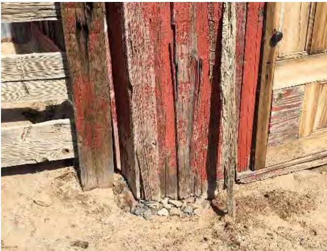
Scott pulling dirt away from wood and stacking rocks to protect and channel water away from corner of Milk Barn; problem area to be monitored.
