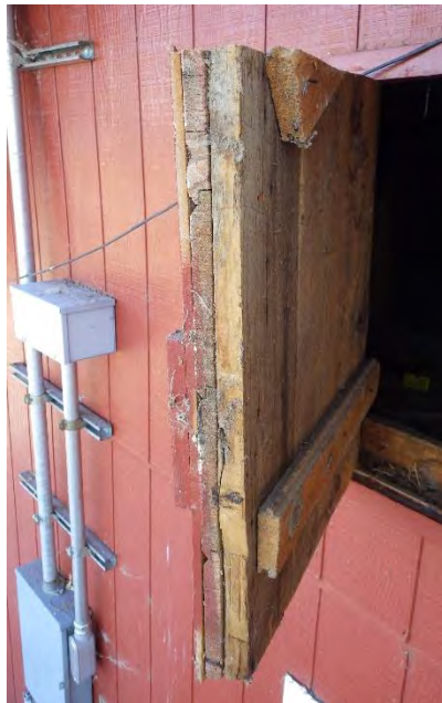
Rt: Entry hatch to oldest mass on the Ranch House; note wood siding under T1-11, appears to run horizontal and be V-grooved; removal of replacement siding would verify historic plus existence of asbestos siding per Gary Bowyer communication
