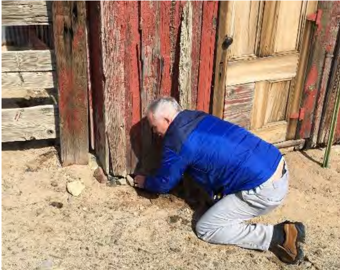
Scott pulling dirt away from wood and stacking rocks to protect and channel water away from corner of Milk Barn; problem area to be monitored.
