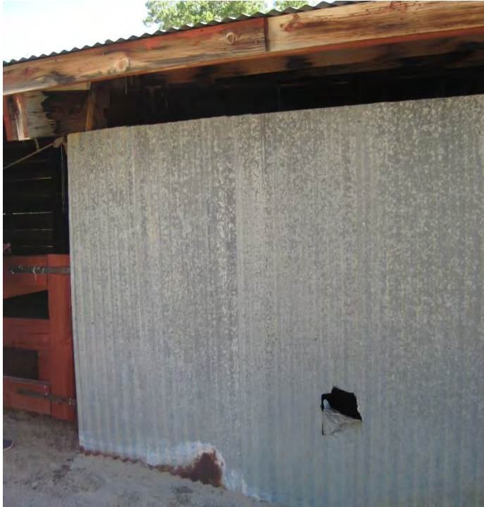
Rust/tears apparent on west wall of Building #8
