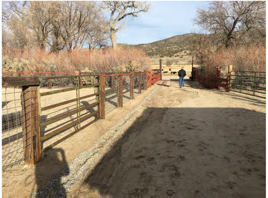
Photo of shallow drain installed to move water towards the Mexican Ditch and away from building foundations and the wood siding on the Milk Barn (December 2018)
