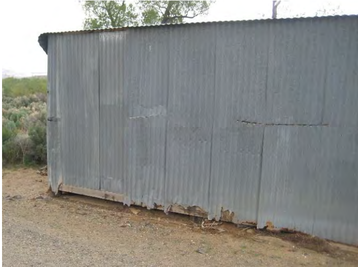
Corrosion occurs when metal sustains ongoing contact with water from snow, rain, and the ground
