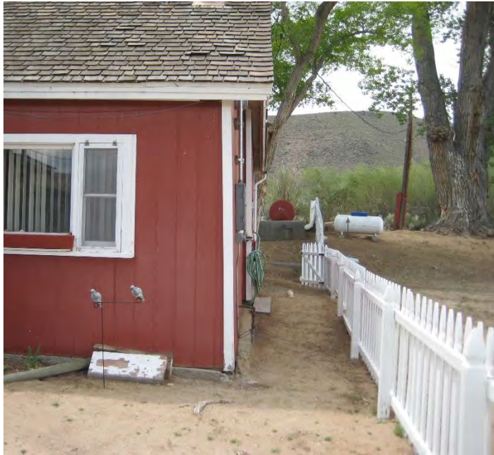
Northeast corner of the residence, view to the west towards the Mexican Ditch; slight inward bowing of north elevation wall of Ranch House is visible suggesting some possible structural concerns; advise a baseline structural assessment that would also include Root Cellar
