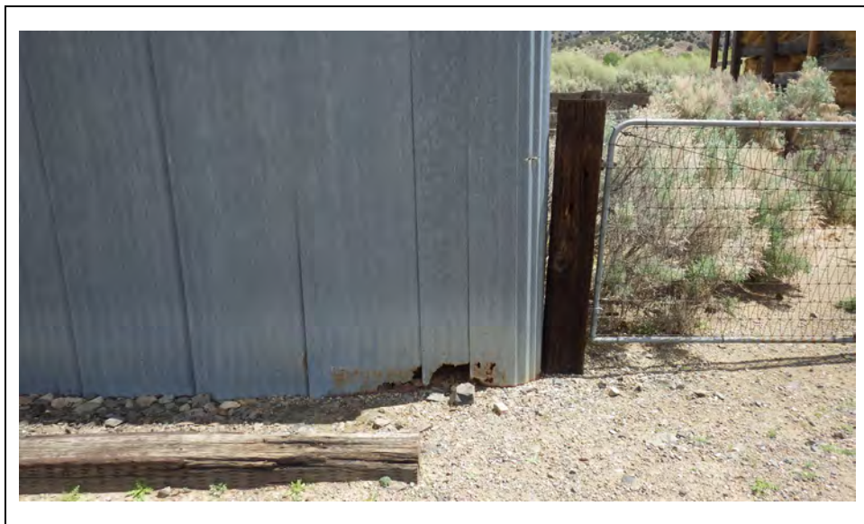
Caption: Feature 6, Southwest corner; detail of damaged corrugated metal sheeting View to: E Photo file name: 1662 Photographer: M. Drews Date: 5/16/2018
