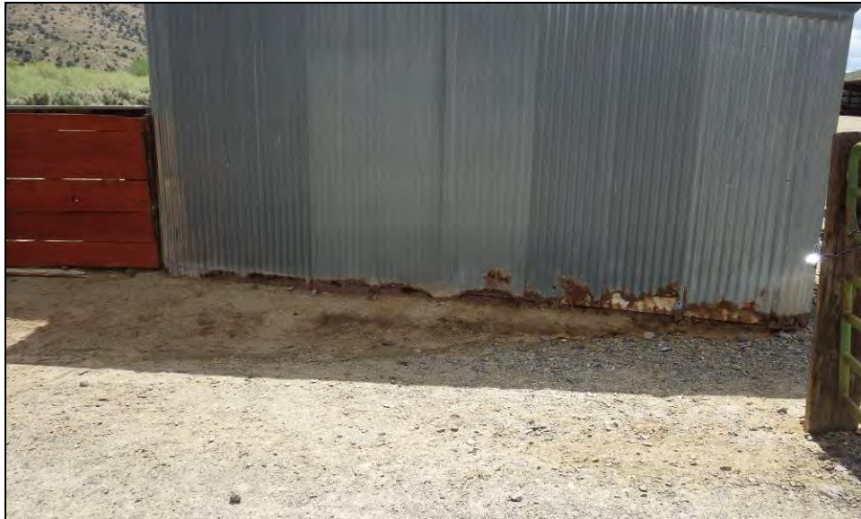
Caption: Feature 6, North elevation; detail of damaged corrugated metal sheeting View to: S Photo file name: 1666 Photographer: M. Drews Date: 5/16/2018
