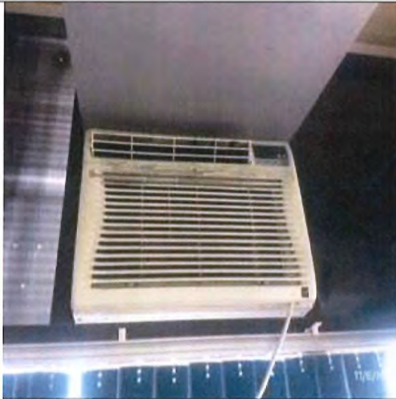
View of Through Wall / Window A/C Unit
