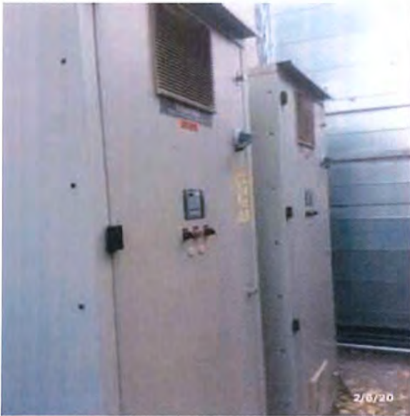
View of Variable Frequency Drive(s) (VFD)
