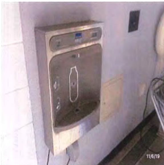
View of Wall Mounted Standard Drinking Fountain with Cooling System (Single)
