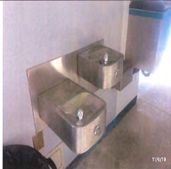
D2018 Drinking Fountains and Coolers :- View of Wall Mounted Standard Drinking Fountain (Dual/Bi-Level)
