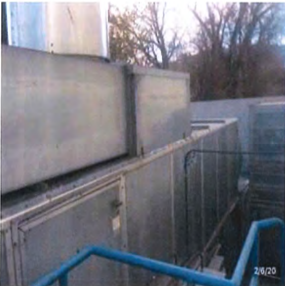
View of Make-up Air Unit - MAU-2
