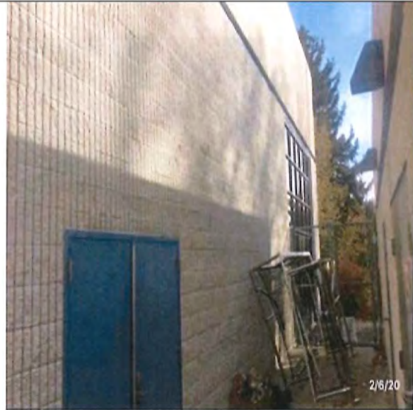
B2011 Exterior Wall Construction :- View of Split Rib CMU Walls
