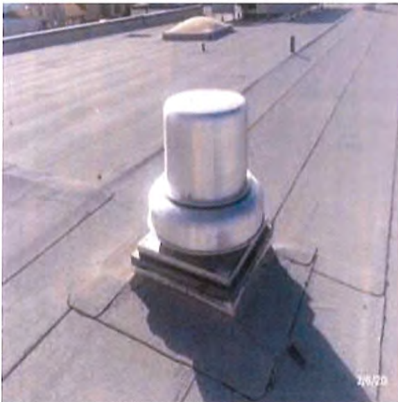
View of Centrifugal Roof Exhaust Fan System
