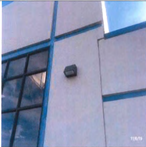
View of Exterior LED Wall Pack Light Fixtures
