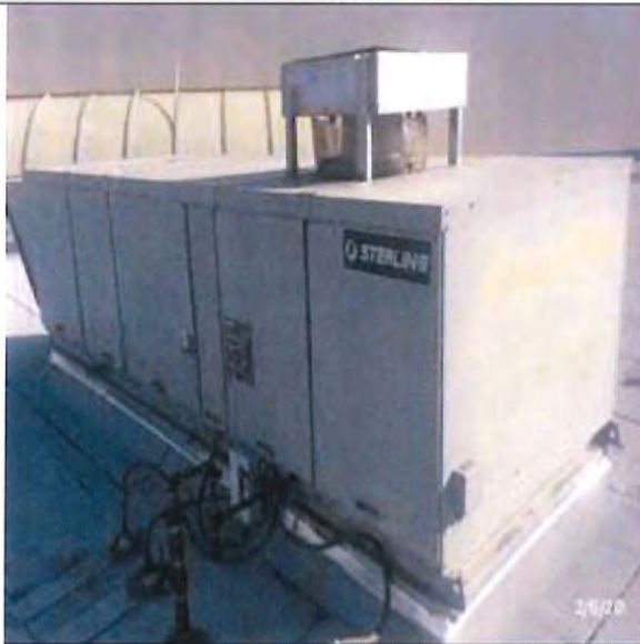
View of Duct Furnace
