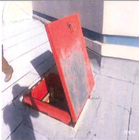
View of Galvanized Steel Hatch
