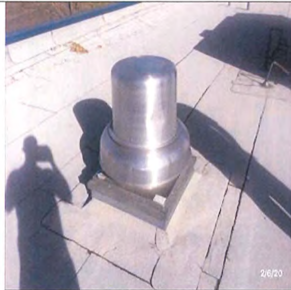
D3042 Exhaust Ventilation Systems :- View of Centrifugal Roof Exhaust Fan System
