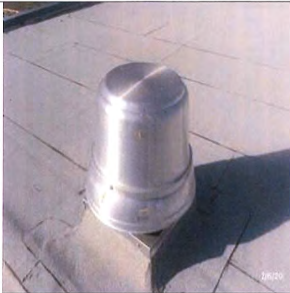
View of Centrifugal Roof Exhaust Fan System
