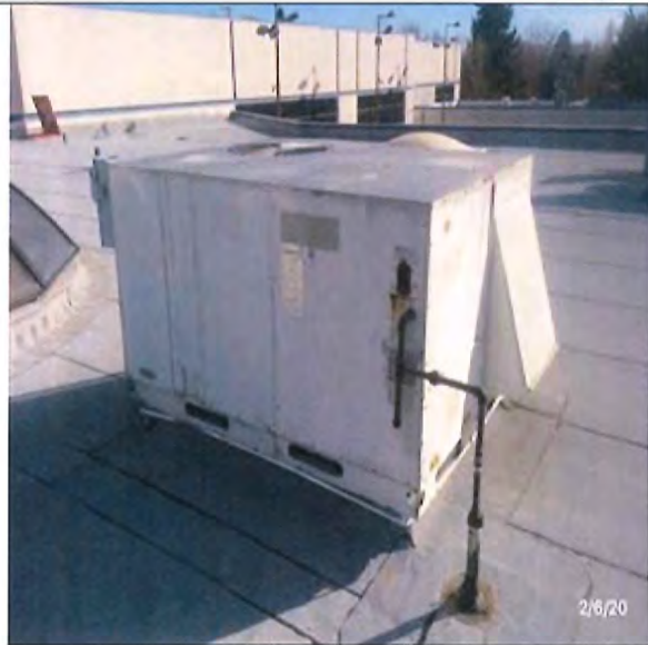
D3052 Package Units :- View of Packaged Rooftop A/C With Heat, Under 20 Tons
