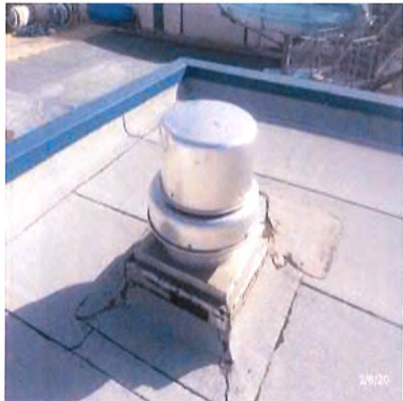
D3042 Exhaust Ventilation Systems :- View of Centrifugal Roof Exhaust Fan System - EF- 1
