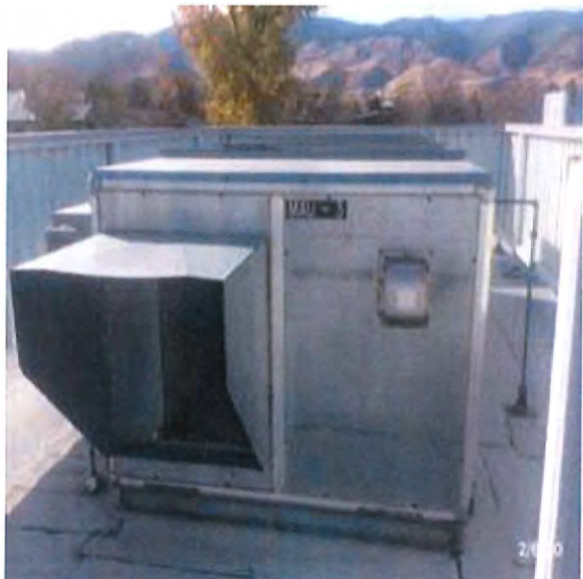
D3041 Air Distribution Systems :- View of Make-up Air Unit - MAU-3
