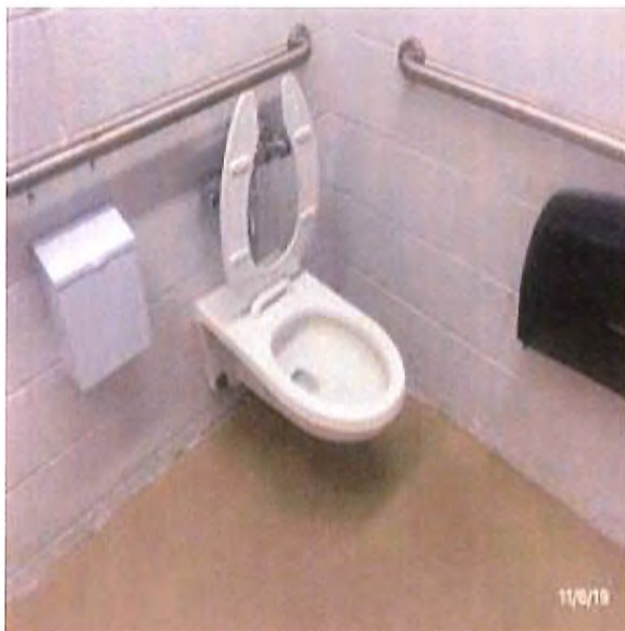
View of Wall Mounted Water Closets
