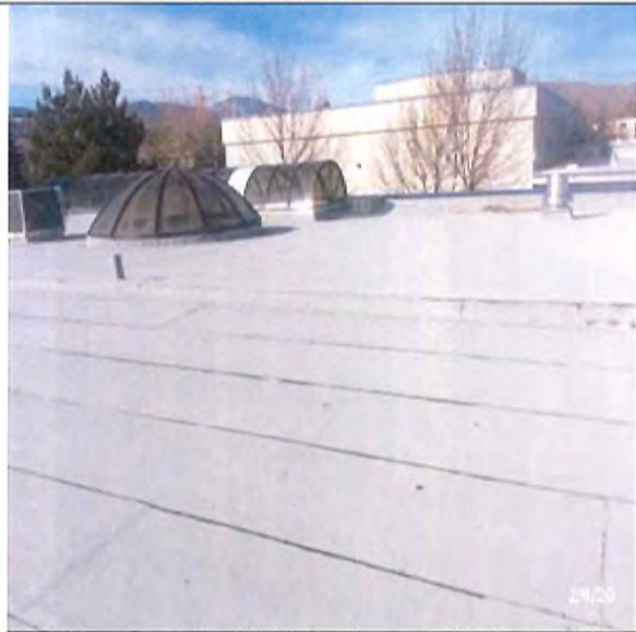
B3011 Roof Finishes :- View of Single-ply Roof Membrane incl. Insulation (Lower)
