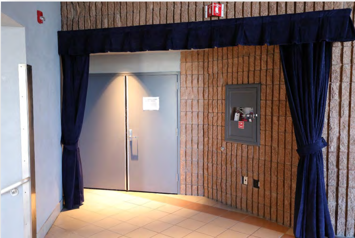
Photo 12 Possible door location to upper ADA seating area – note the recessed fire extinguisher cabinet and electrical outlets that will have to be relocated
