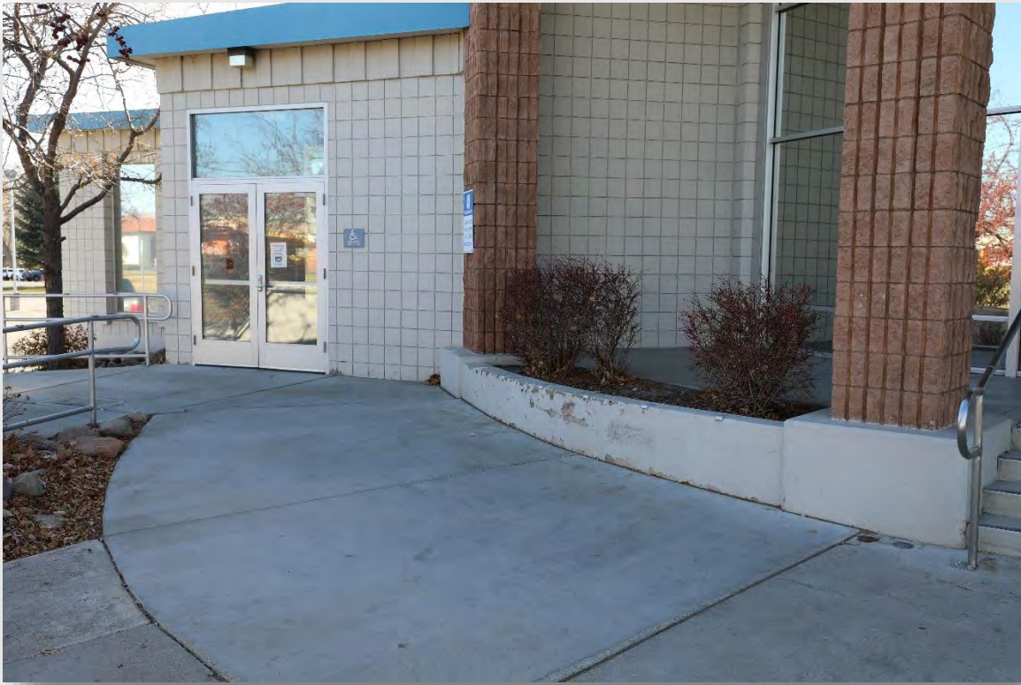
Photo 7 Running slope in direction of travel exceeds 5% and should be considered a ramp with level landings top and bottom and handrails on both sides
