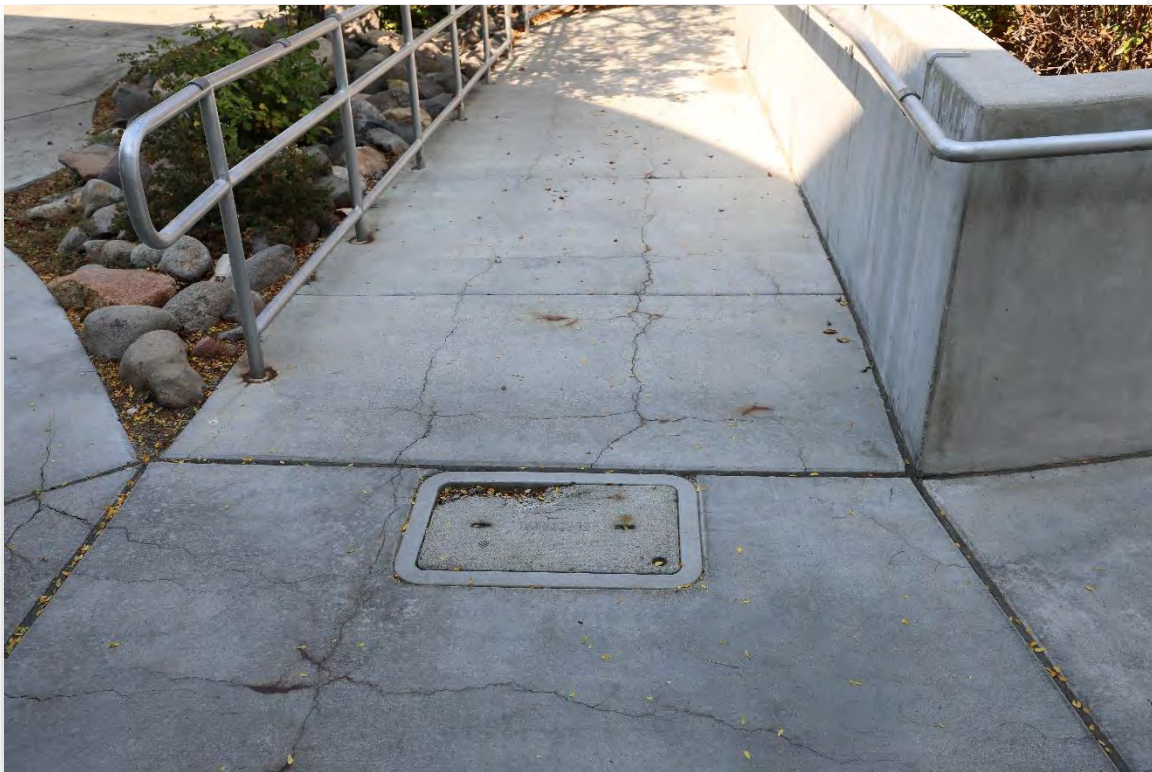
Photo 6 damaged vault lid in accessible route at east ramp looking north
