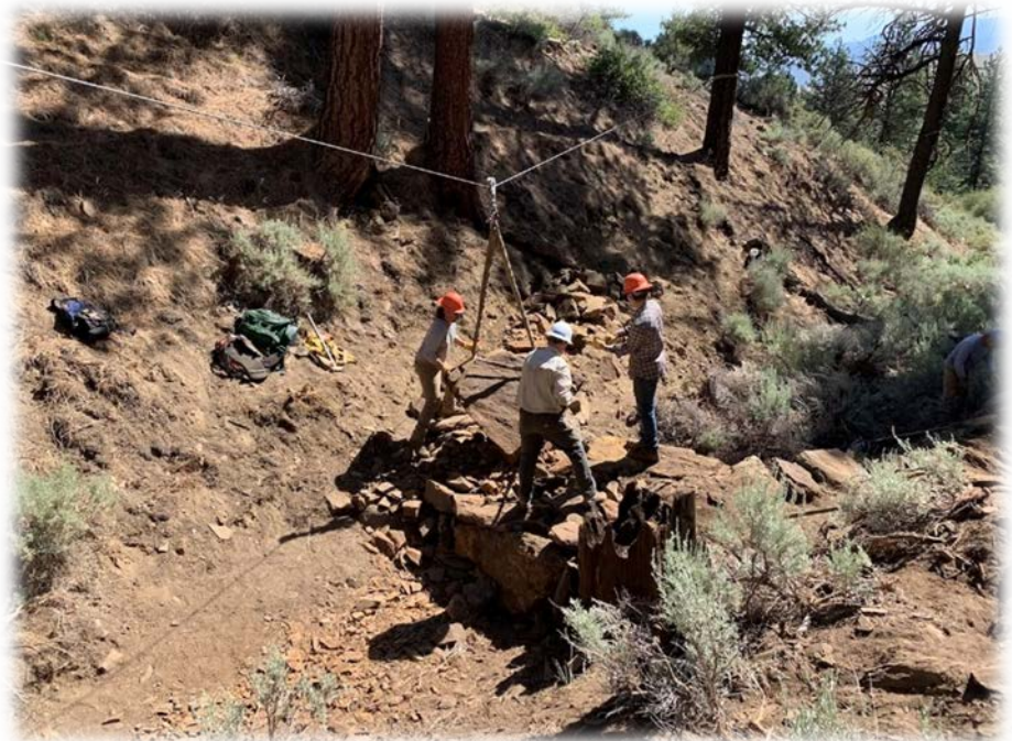
Rock bridge construction on Lincoln Bypass
