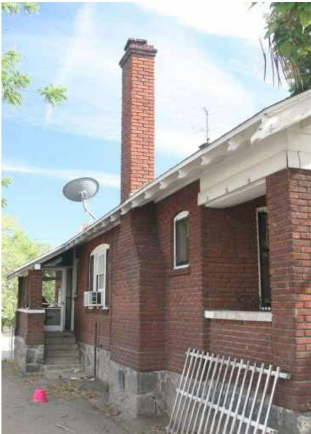
**Figure 19.** Unreinforced masonry residence. The home is built on an inhomogeneous rubble-rock foundation, is likely not tied to the foundation, is made of ridged brick that break apart with strong earthquake forces, and has a topple hazard, the tall chimney. Possible secondary hazards include gas leaks and fire if the gas meter or hoses are damaged or further damaged by aftershocks. Shelter would likely be required for the residents following a major earthquake.
