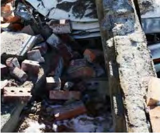
**Figure 21.** Bricks and crowning bond beam that fell on a car during the 2008 Wells, Nevada earthquake. Unreinforced masonry buildings can shed debris like this on sidewalks, alleys, and other buildings around them.
