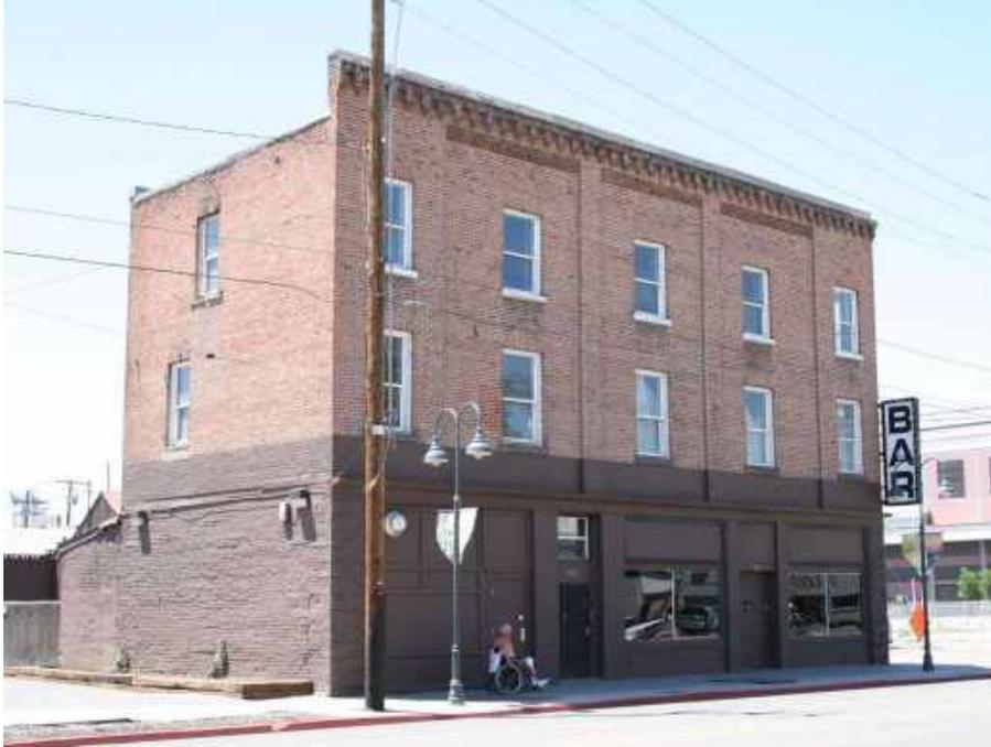
**Figure 20.** Unreinforced masonry commercial building with an unsupported parapet and crowning bond beam. The wheelchair-bound man below would have a difficult time getting out of the way during the shaking from an earthquake.
