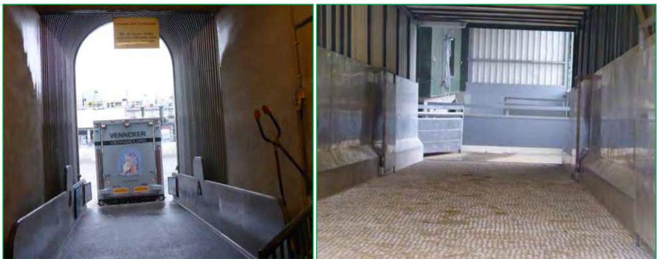
Make the sides of the loading ramp high and solid
