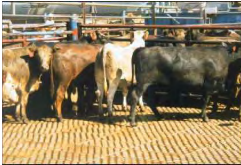
A good sample of non-slip flooring
