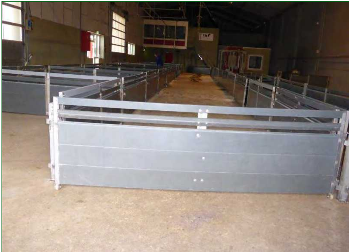
Export station Harfsen uses plastic fencing. Because of this, there is hardly any noise in the lairage.
