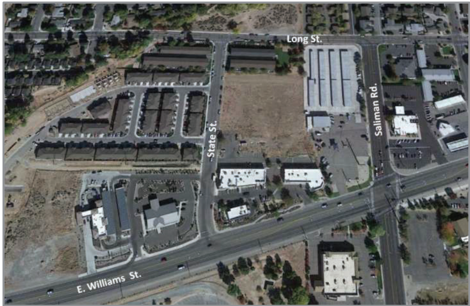
Figure 10: Existing State Street Intersection (Source: Google)
