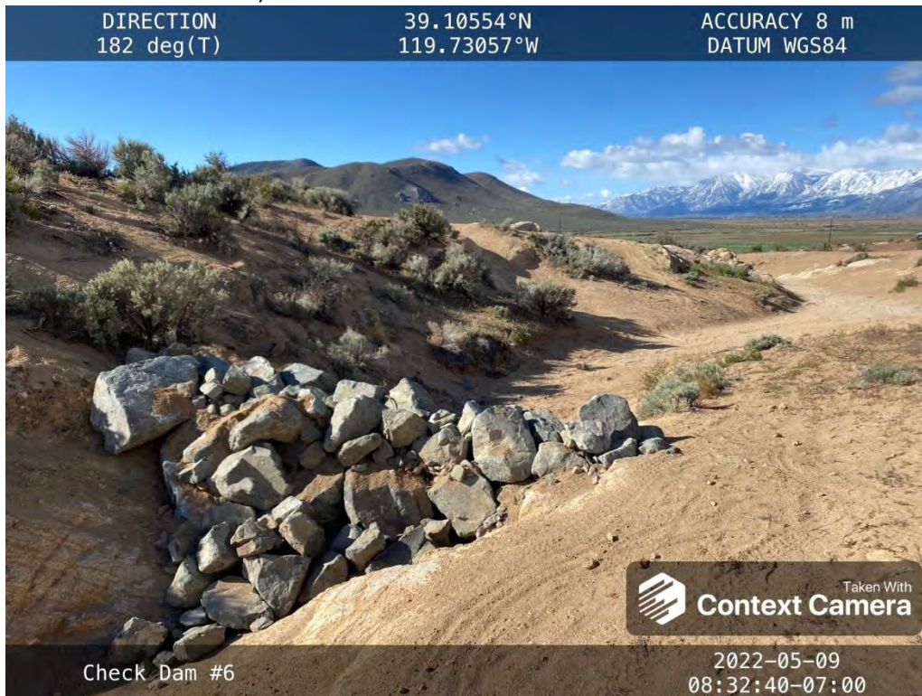
2022 Condition, Post-Construction – New check dam to slow flows
