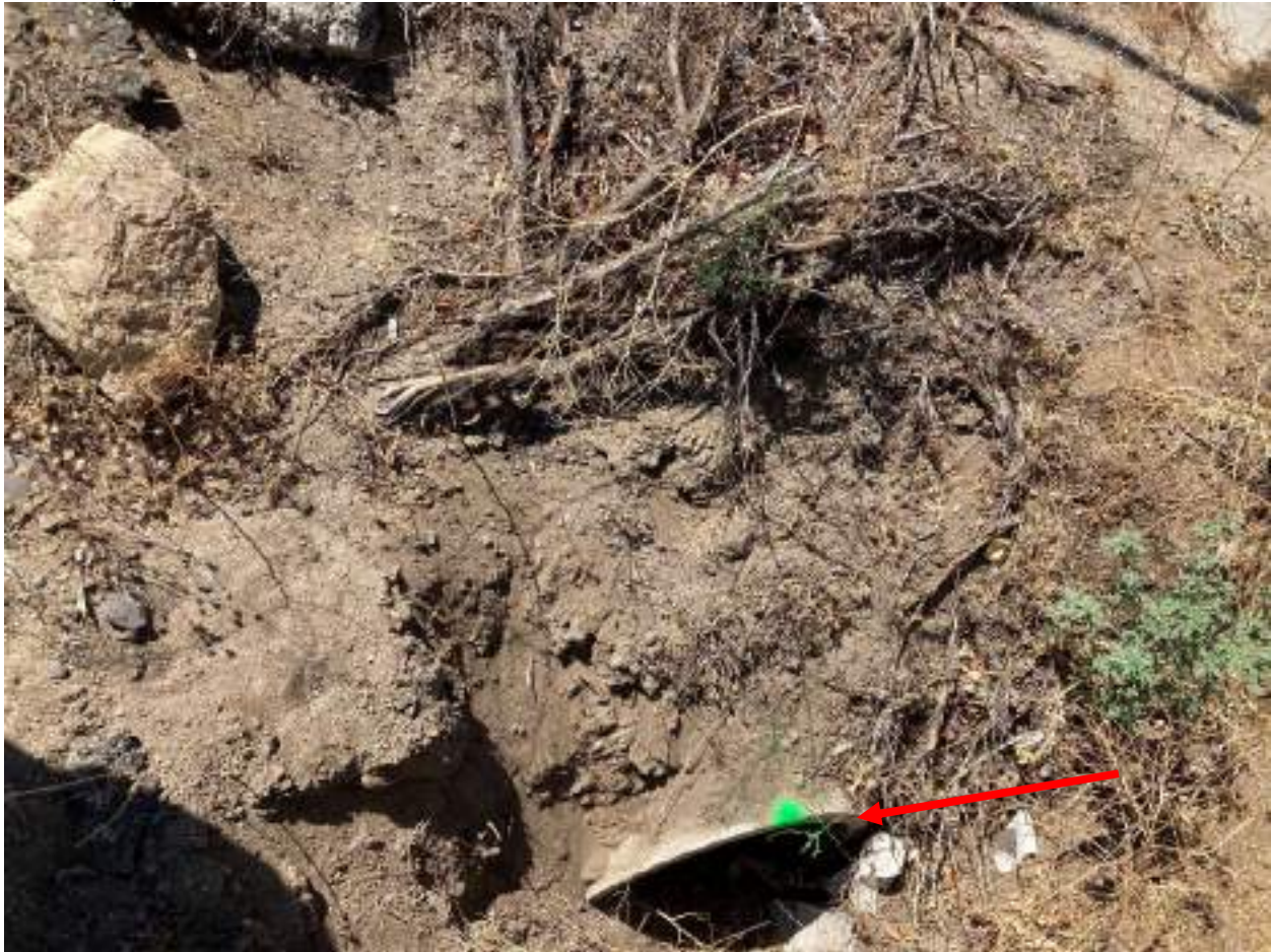
Figure 5 – Buried 15” RCP which daylights and extends south into Medical Pkwy. The entrance to the RCP is mostly buried (approximately 2/3rds) by sediment and debris. This RCP will need to be cleared of debris in order for it to function properly.
