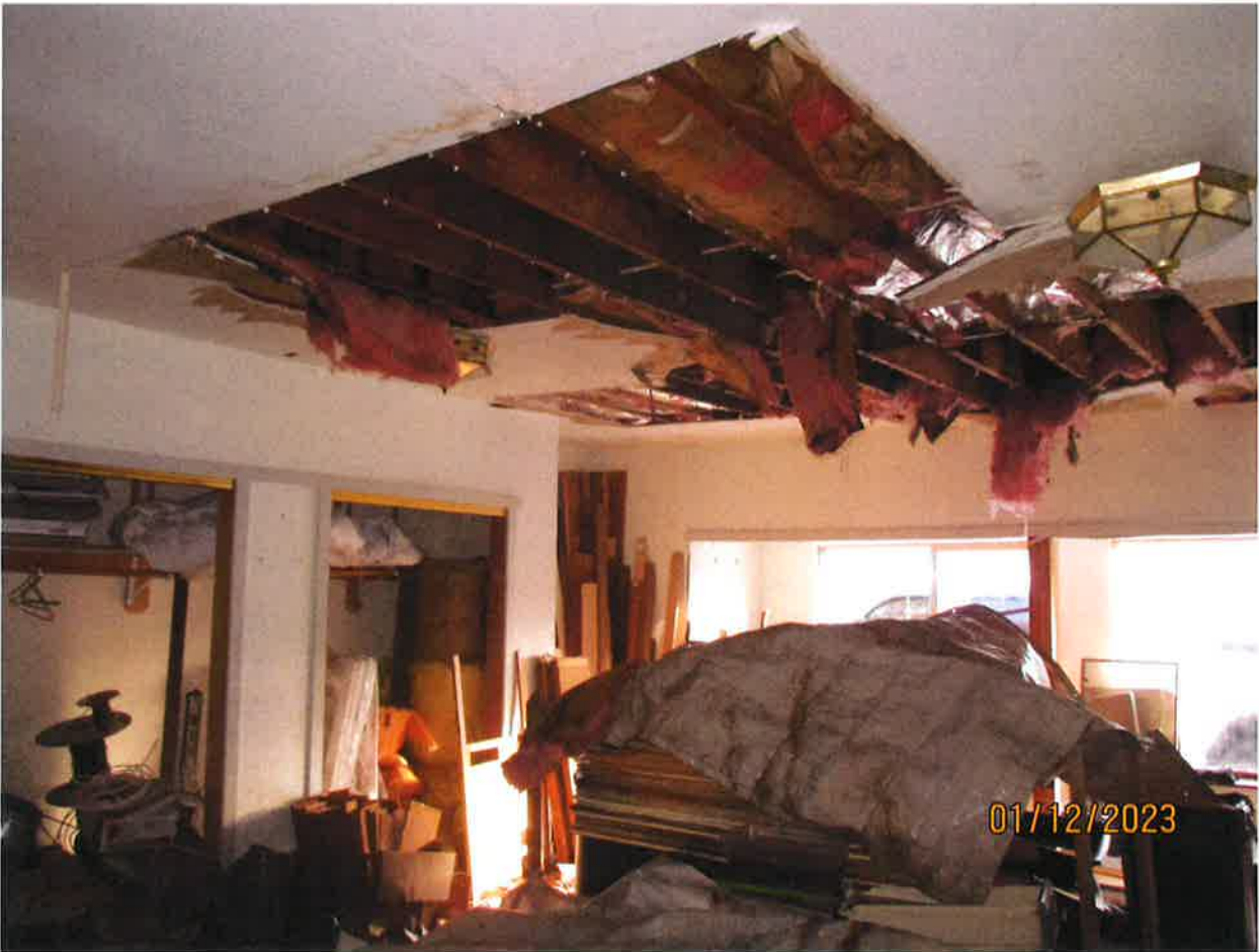
Converted Garage Ceiling
