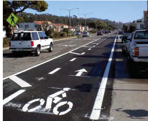
The use of additional pavement markings delineates space between vehicles and cyclists.
