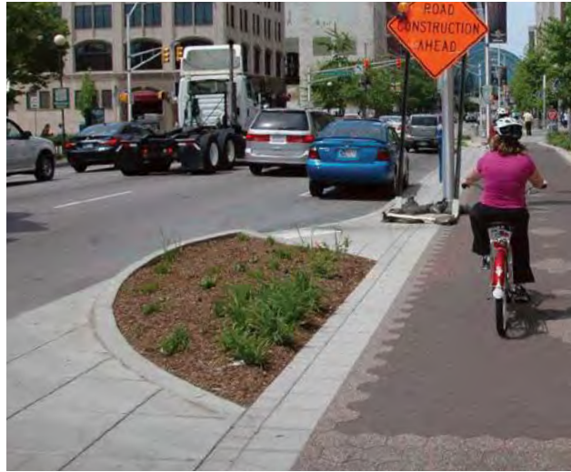
Raised separated bikeways are bicycle facilities that are vertically separated from motor vehicle traffic.
