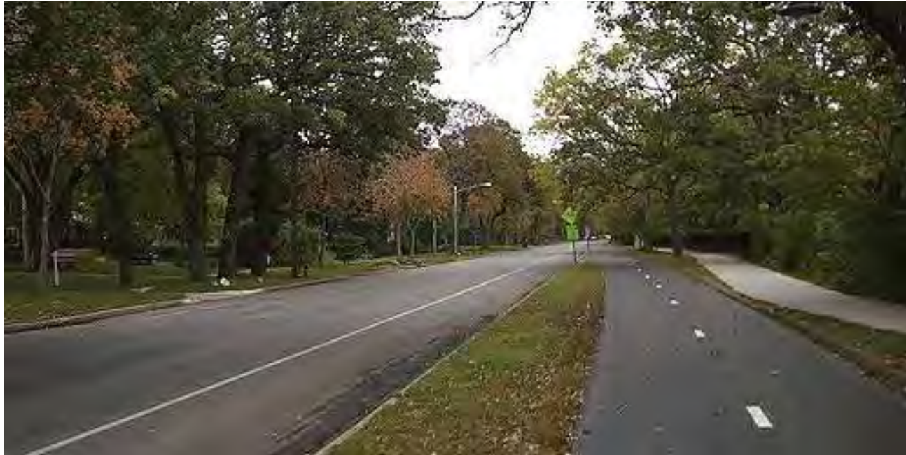
A sidepath provides a continuous path of travel along roadway corridors with few driveways or intersections. Depending on the anticipated volumes and context, the sidepath can be constructed in lieu of sidewalk and/or bike lanes. Oftentimes, anticipated volumes, mix of skills, or other factors such as route continuity will also be considered in the decision to also include bike lanes and sidewalks.
