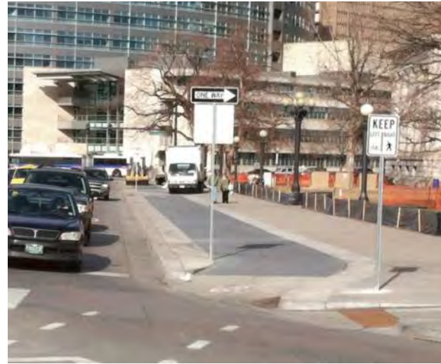
Raised separated bikeways are bicycle facilities that are vertically separated from motor vehicle traffic.
