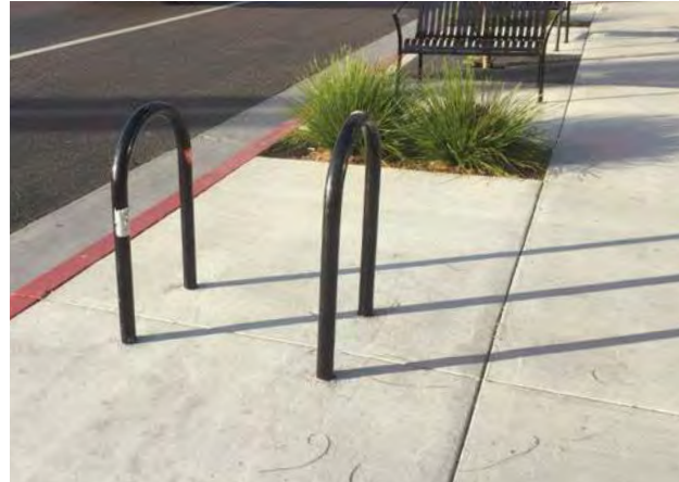
Inverted-U racks provide two points of contact.
