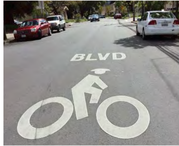
An example of a large pavement marking to reinforce that the street is a Bike Boulevard.
