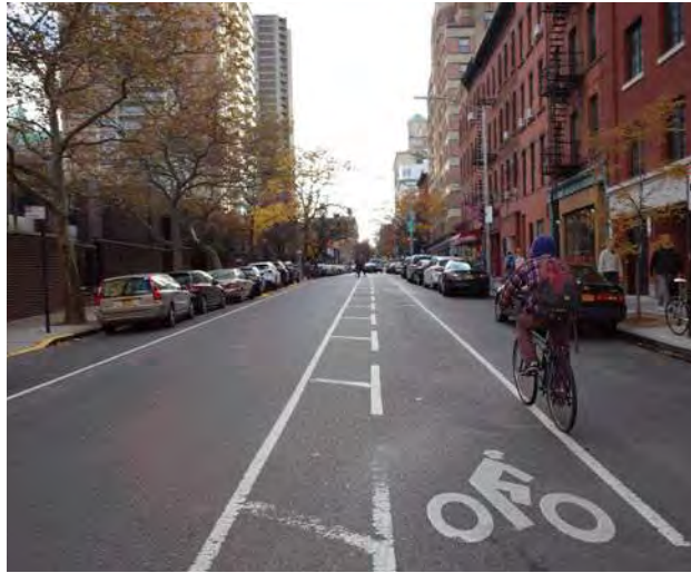
Buffered bike lanes should consider both vehicular traffic and parked cars.
