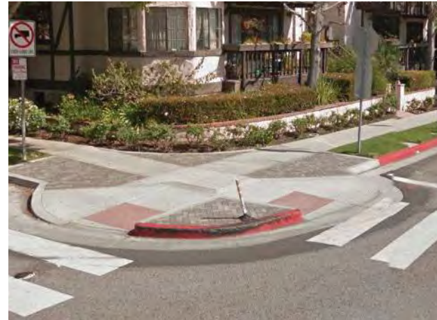
Recommended: Bulb-Out with bidirectional curb ramps for crossing in both directions. Source: Google Streetview
