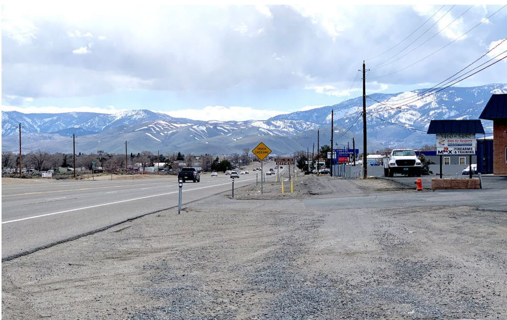
Sections of multiuse path on US 50 do not have clear delineation between shoulders and access driveways.
