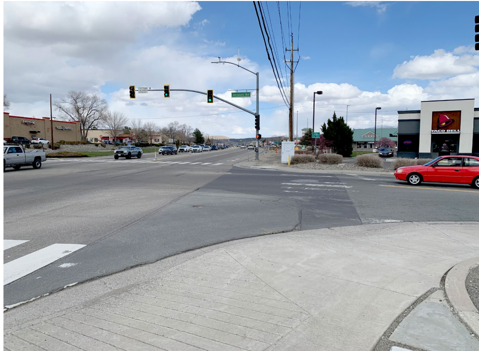
Intersection of US 50 and Airport Road. Inconsistent sidewalk, faded crosswalk, gap in connectivity.
