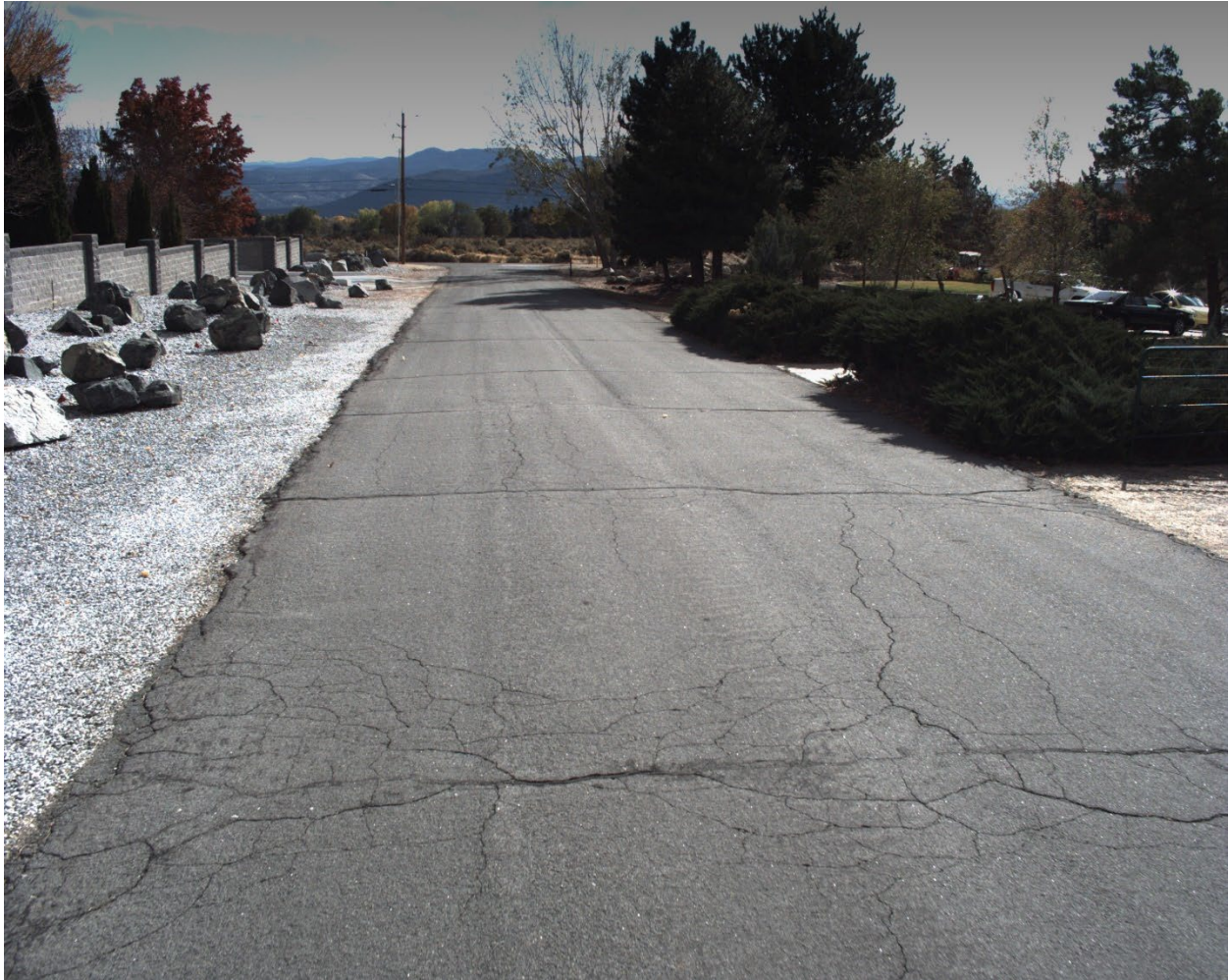
Figure 8. Pavement in Poor condition category (PCI 55–41).
