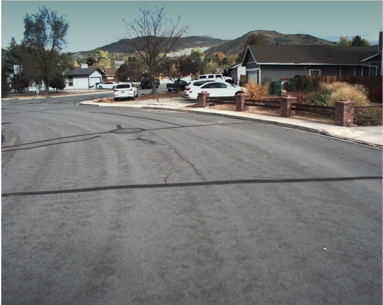
Figure 6. Pavement in Satisfactory condition category (PCI 85–71).
