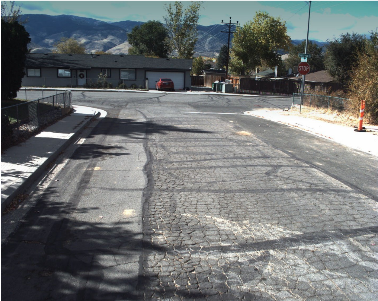
Figure 10. Pavement in Serious condition category (PCI 25–11).
