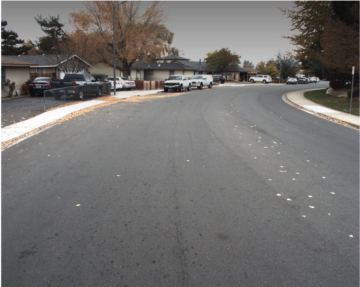
Figure 5. Pavement in Good condition category (PCI 100–86).
