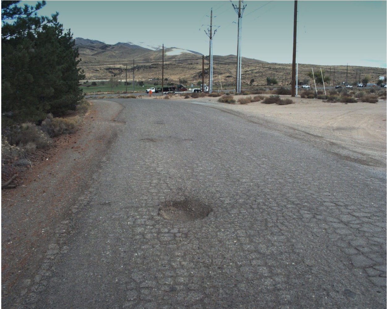
Figure 11. Pavement in Failed condition category (PCI 10–0).
