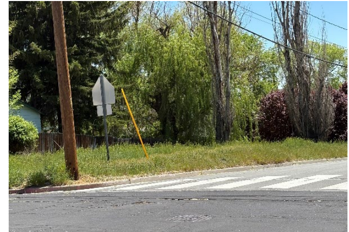
Figure 29: Missing curb ramps and sidewalks across N Fall St at the intersection of Corbett St.
