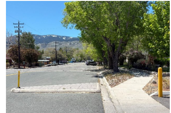
Figure 36: Concrete islands on E John St.
