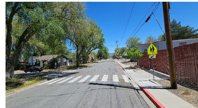
Figure 32: Crosswalk across E Park St that leads to N Peter's St that has no curb ramps or sidewalks.
