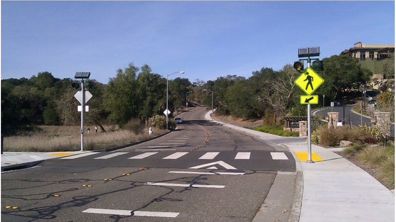
Raised pedestrian crossings help reduce vehicle speeds and give pedestrians greater prominence as they cross the street.
