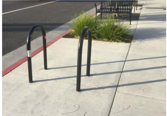
*Inverted-U racks provide two points of contact.*
