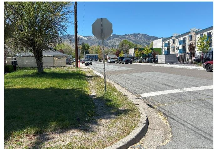
**Figure 30: Missing curb ramps and sidewalks across N Fall St at the intersection of E Park St.**
