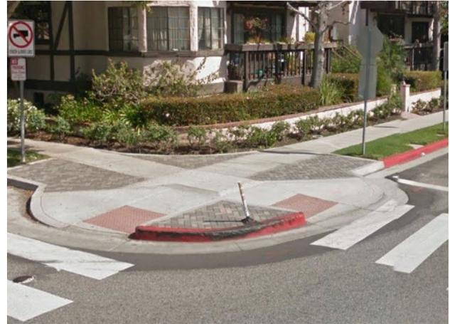
*Recommended: Bulb-Out with bidirectional curb ramps for crossing in both directions. Source: Google Streetview*
